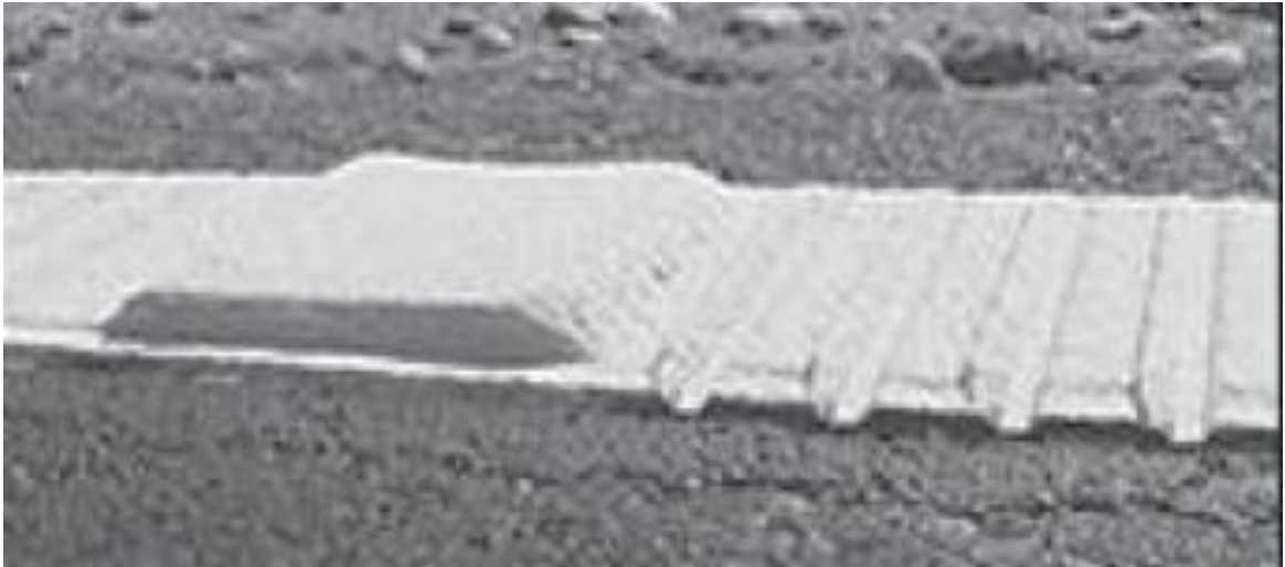
Exhibit 4.1 – Raised Audible Pavement Marking:
