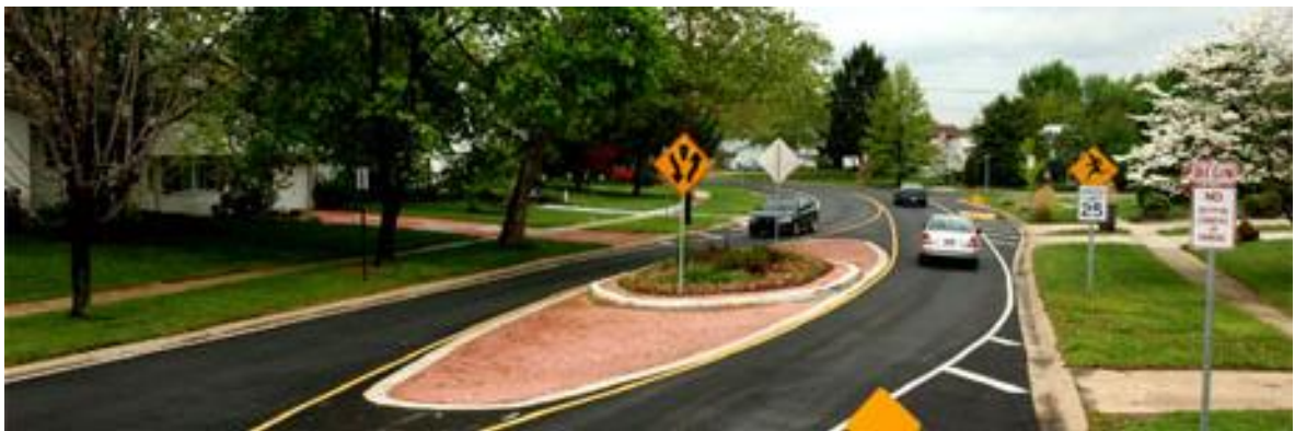
Exhibit 3.7 - Typical Center Island Narrowing Application:
