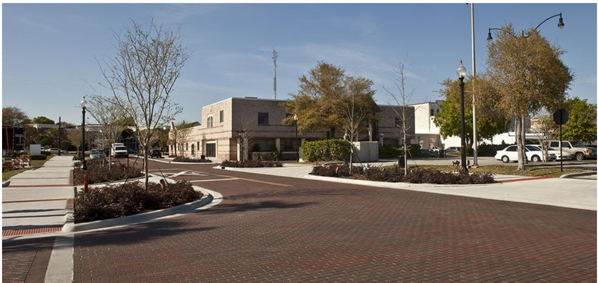
Exhibit 3.4 - Typical Textured Pavement Application: (clay brick pavers shown)
