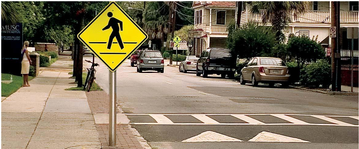
Exhibit 3.2 - Typical Speed Table Application:
