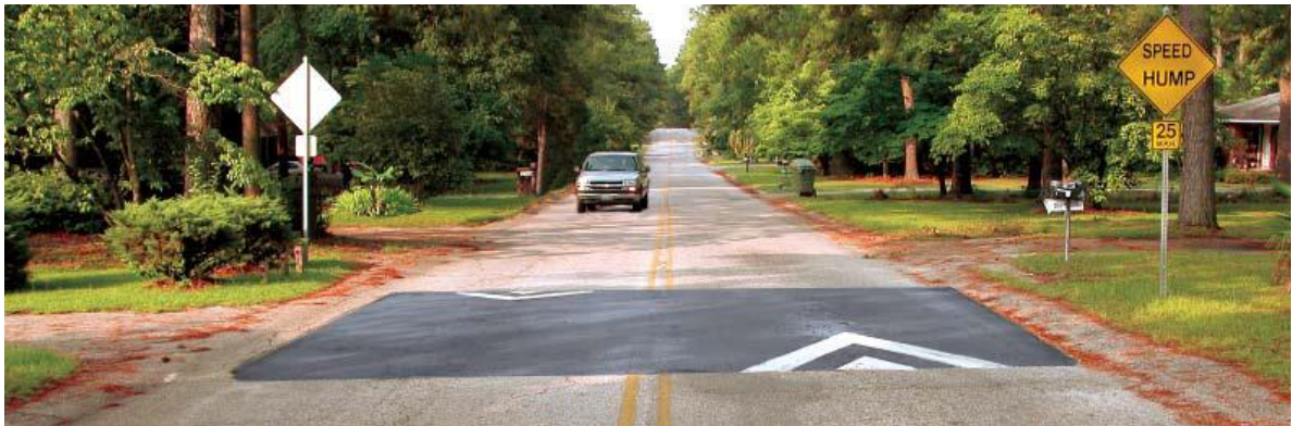
Exhibit 3.1 - Typical Speed Hump Application:
