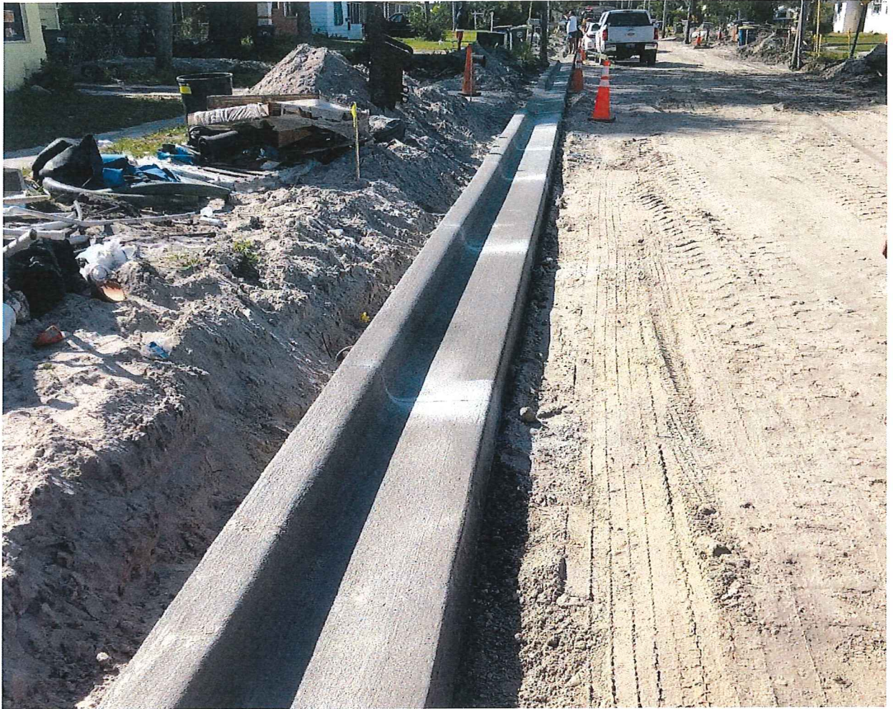
Curb and Gutter Installation
