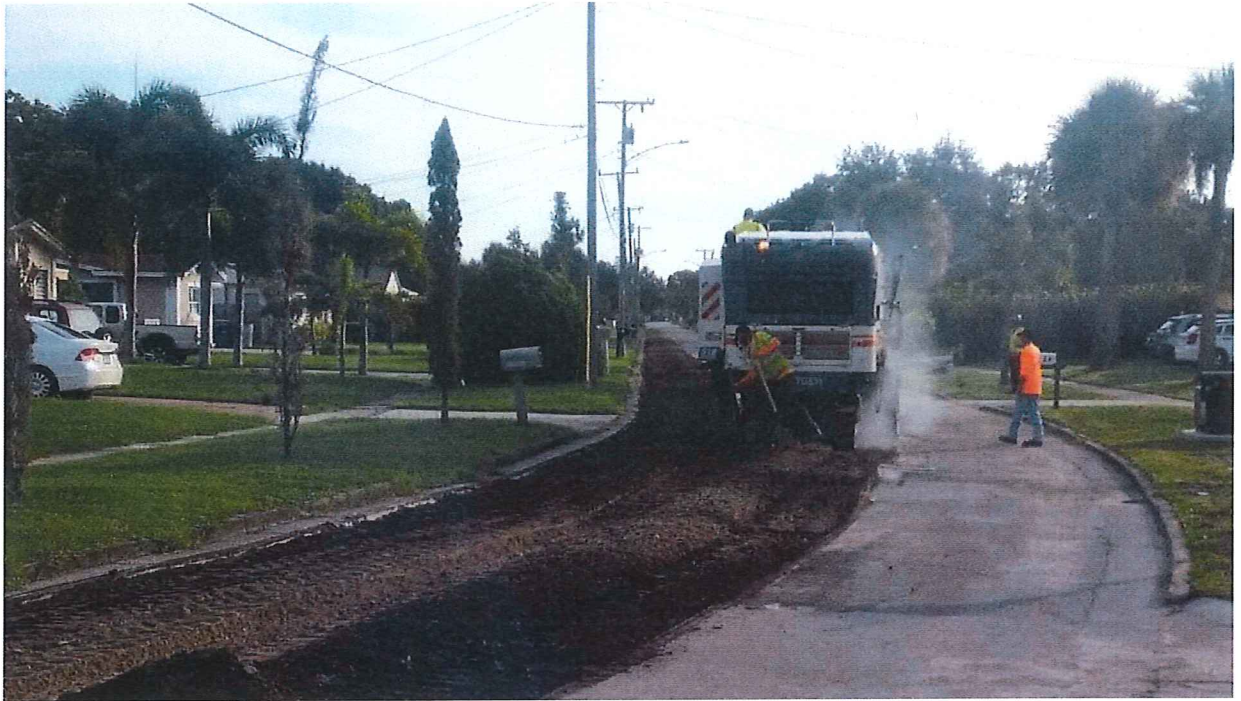
Milling Old Roadway Surface
