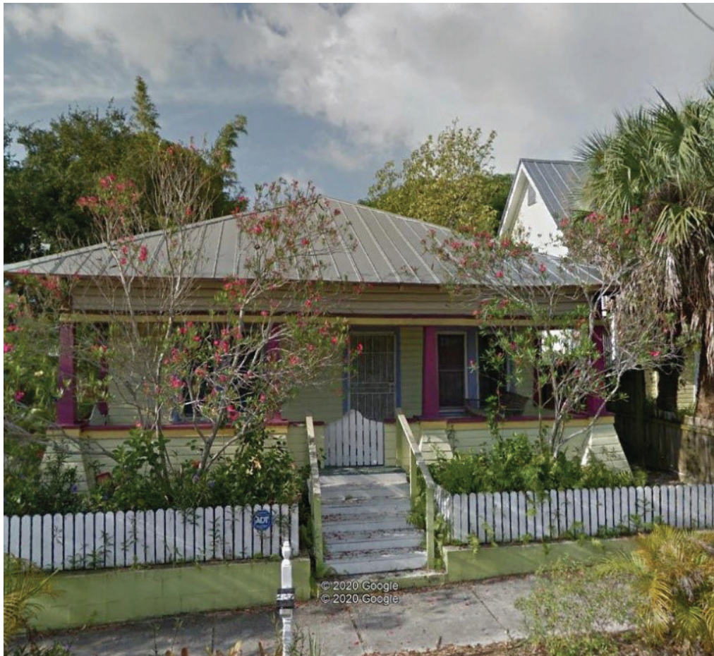
207 Avenue D - Previous Condition
