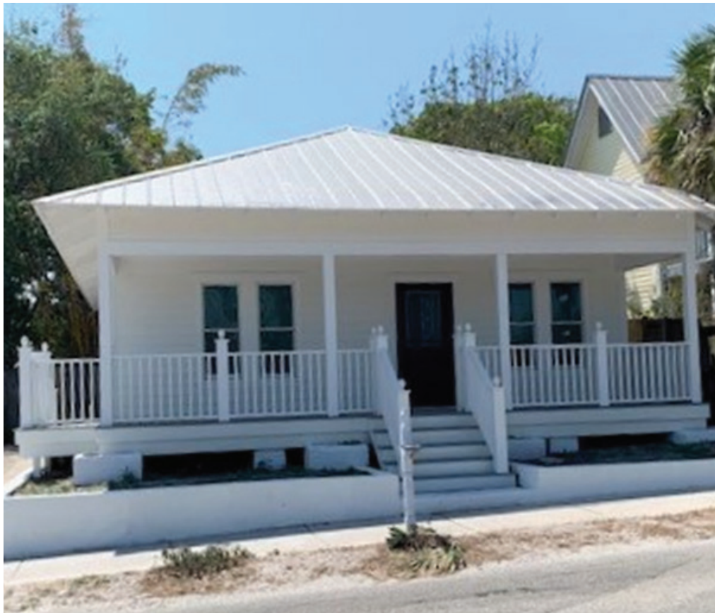
207 Avenue D - Current Condition
