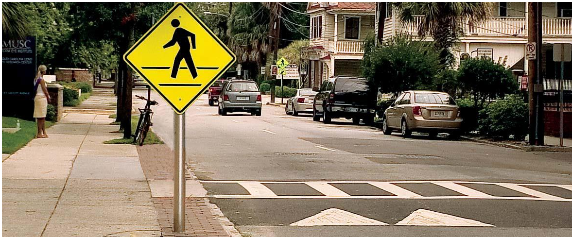
Exhibit 3.2 - Typical Speed Table Application:
