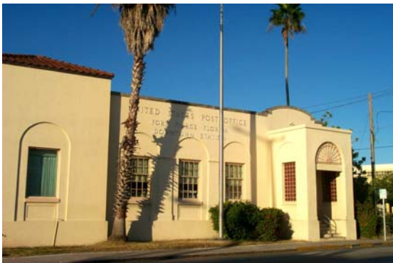
The Fort Pierce Post Office on Orange Ave.
