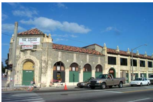
Intersection of US 1 and Orange Ave.
