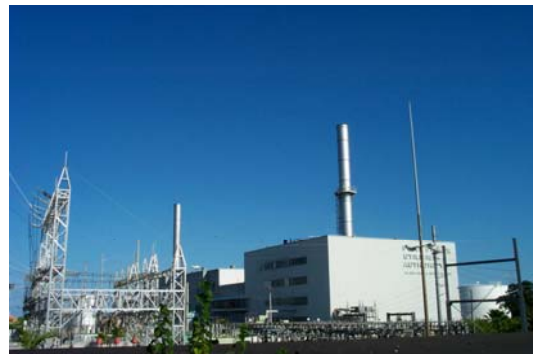
Fort Pierce Power Plant
