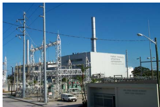
The Fort Pierce Power Plant in 2001
