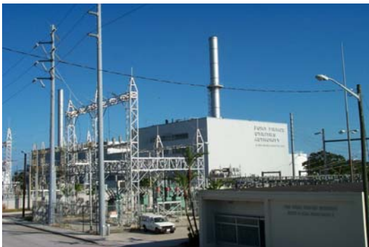
Fort Pierce Power Plant
