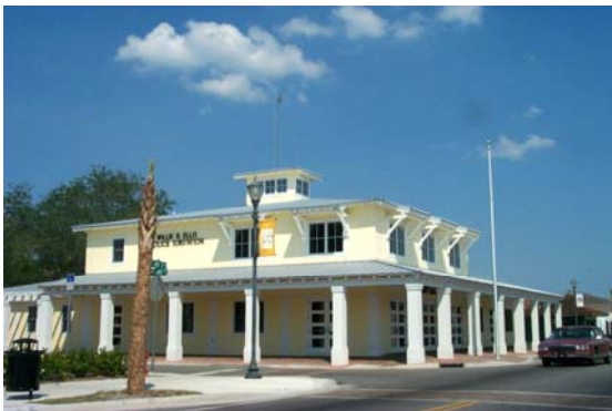
Police Substation on Avenue D
