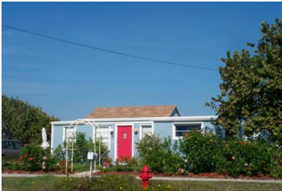
Typical older beach house on SR A1A Drive
