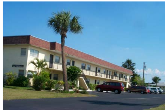
Typical older condominium off Seaway
