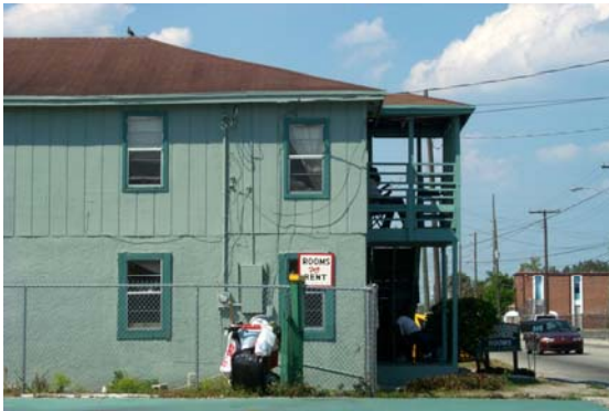
Multifamily structure off Avenue D
