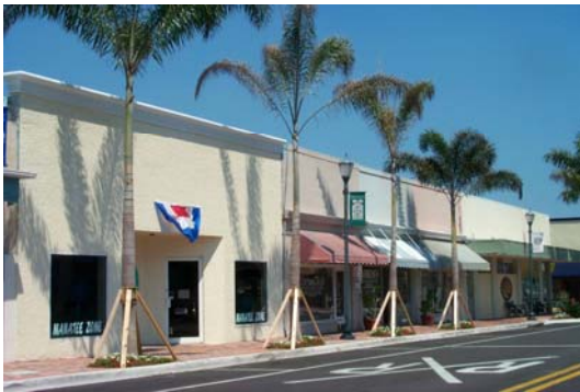
Orange Avenue Improvements, 2001
