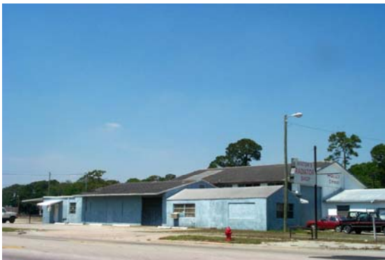
Typical commercial on Orange Ave. at 33rd
