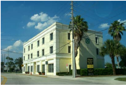
Restored office building on Indian River Drive
