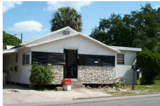
Altered historic house on Avenue B
