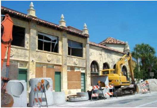
Orange Avenue under construction in 2001
