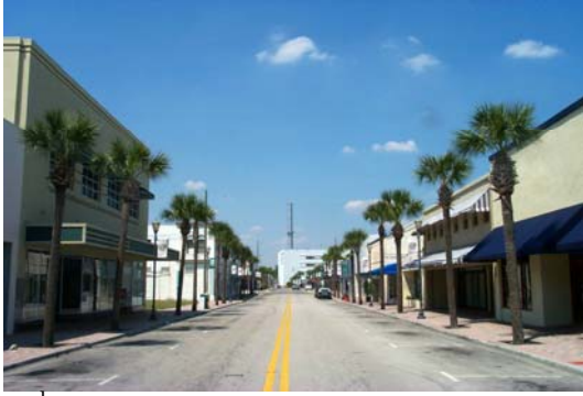
2 nd Street Improvements in 2001
