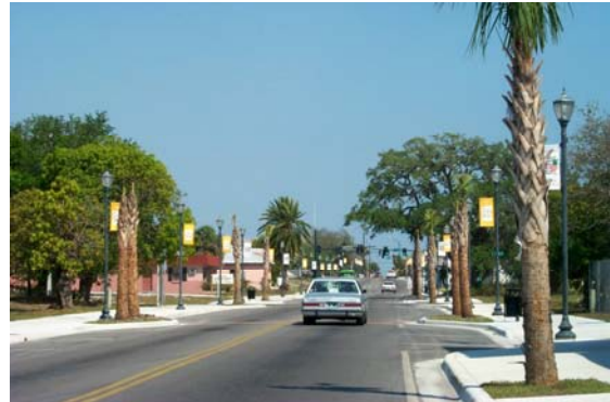
Avenue D improvements
