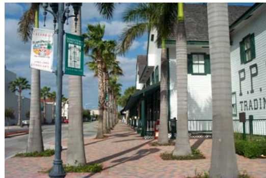
Buried lines on Orange Avenue
