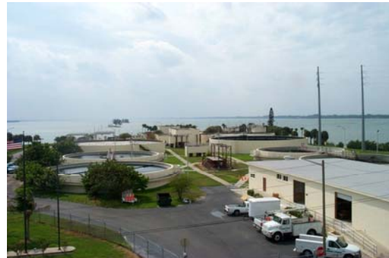
The regional water reclamation facility
