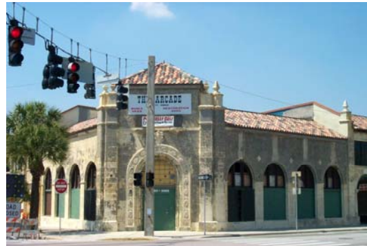
The Arcade under construction in 2001
