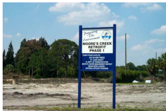
Moores Creek improvement project
