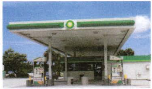
Gas Station Under Development | Port Saint Lucie
