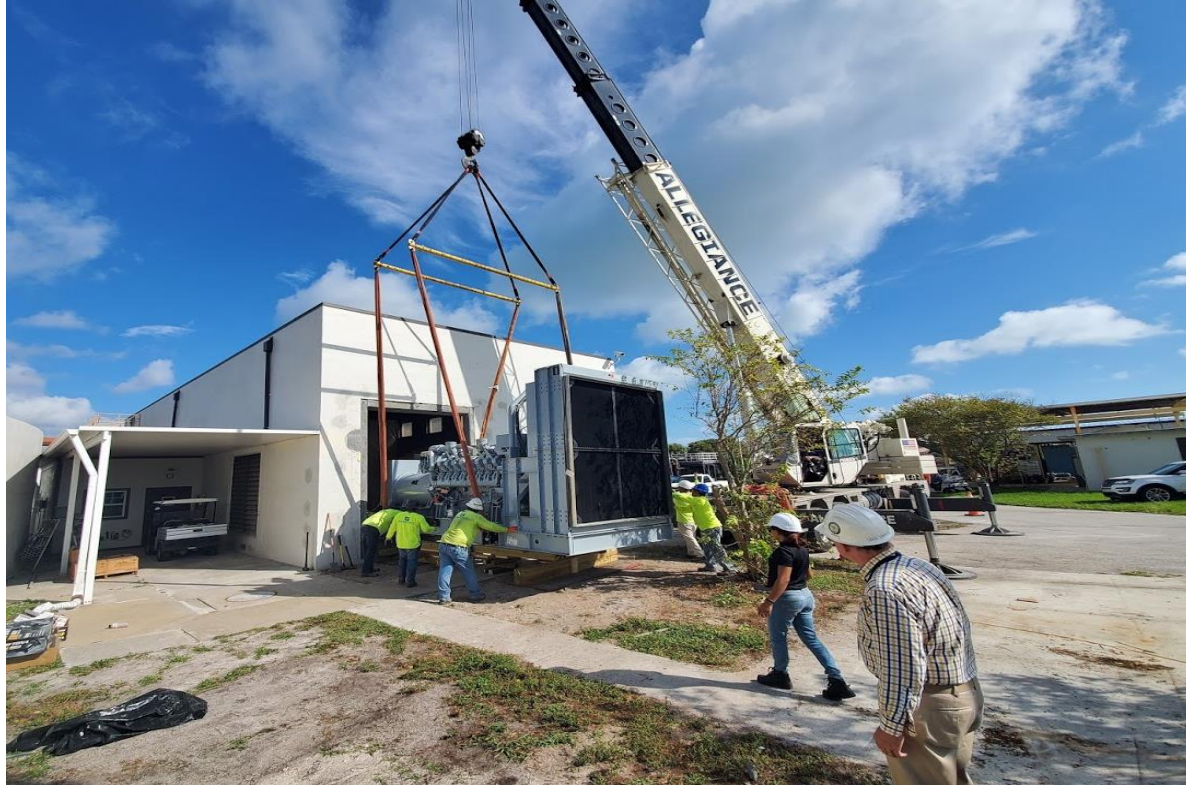
Generator on slide ramp, methodically being pushed into the blower room.
