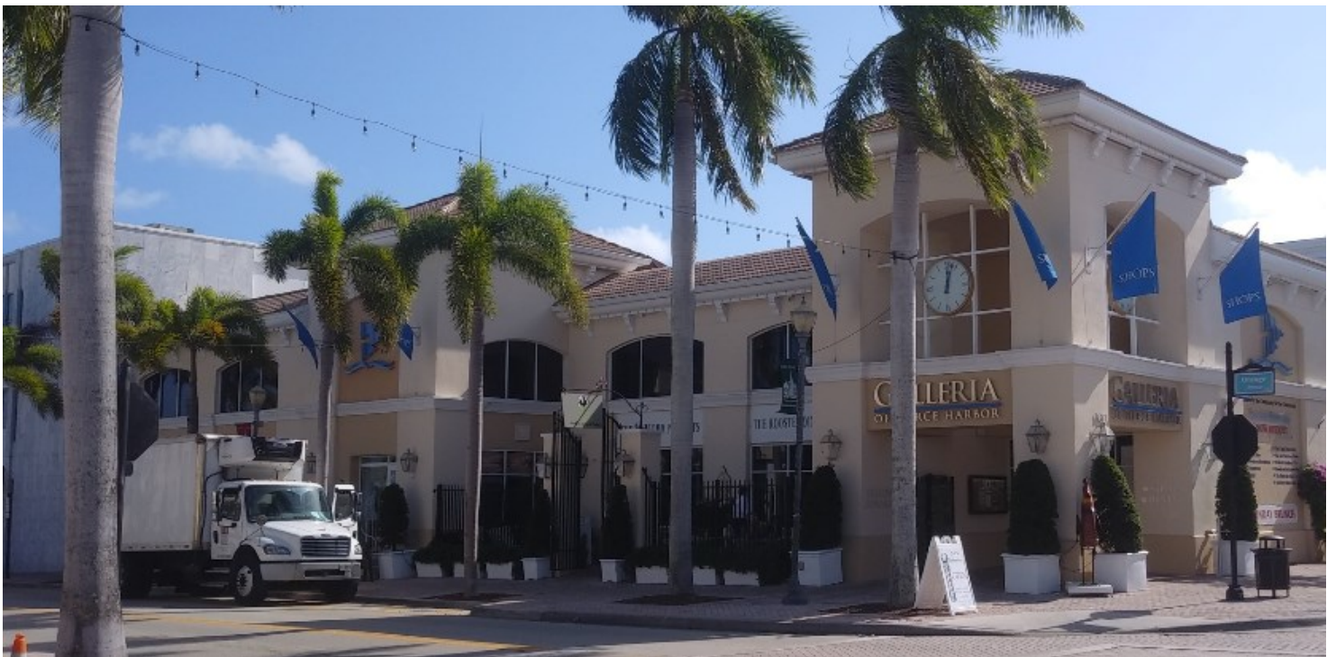
Current Orange Avenue façade
