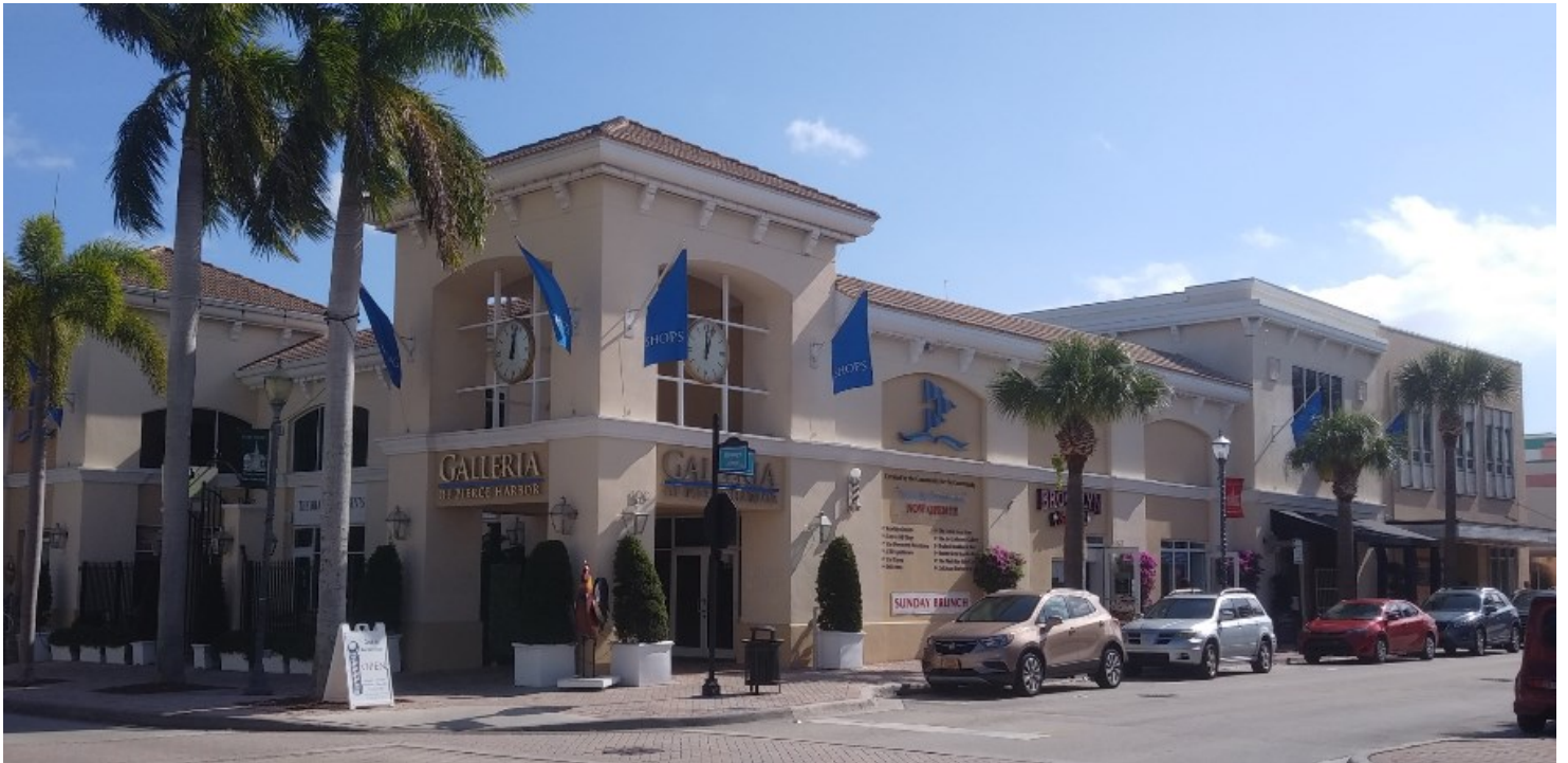
Current South 2nd Street façade
