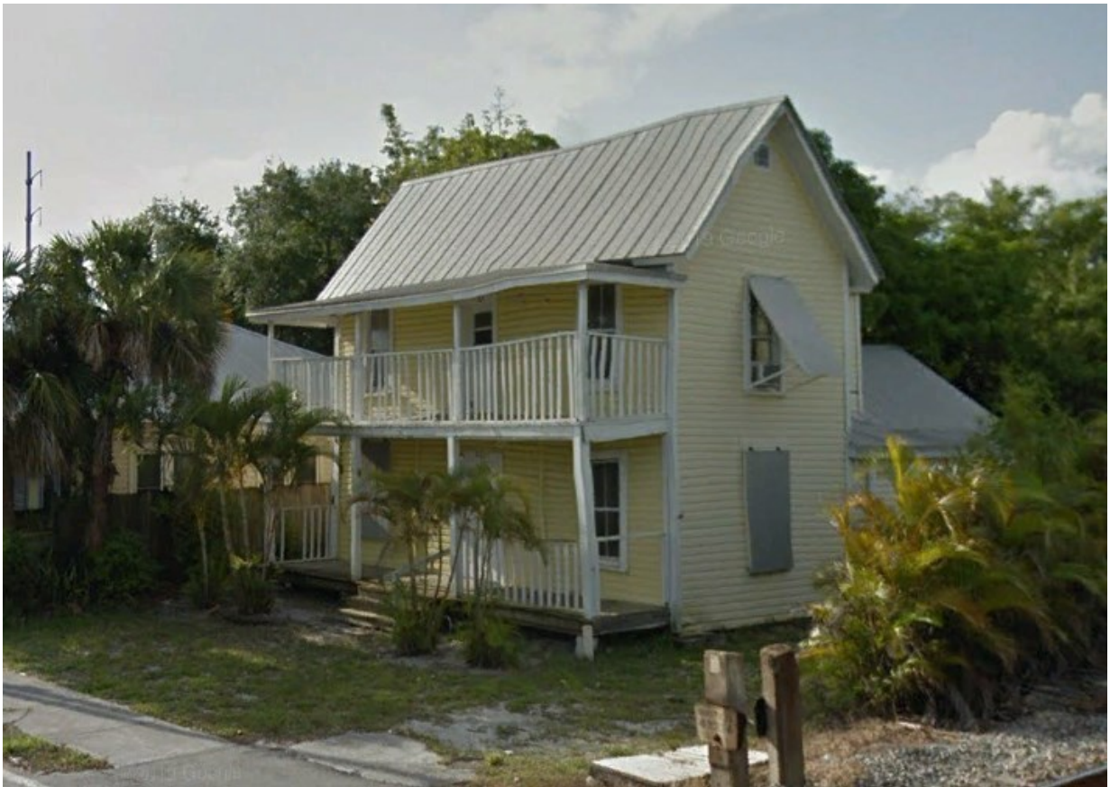
Current Building Conditions
