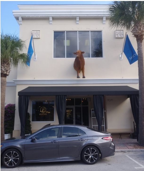
Existing southwest facade
