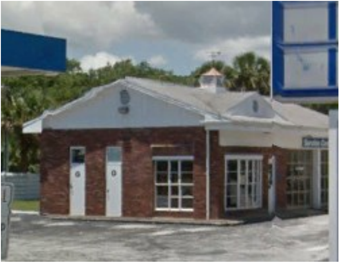
EXISTING NORTHEAST FAÇADE
