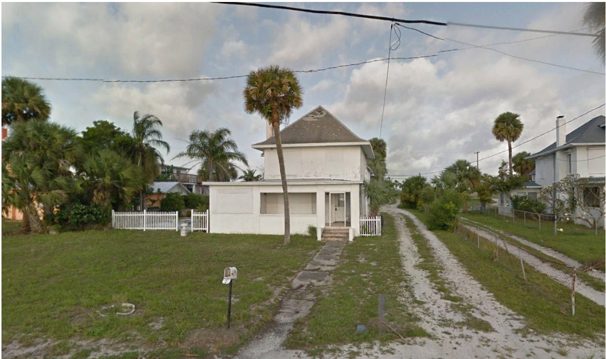
Indian River Drive façade
