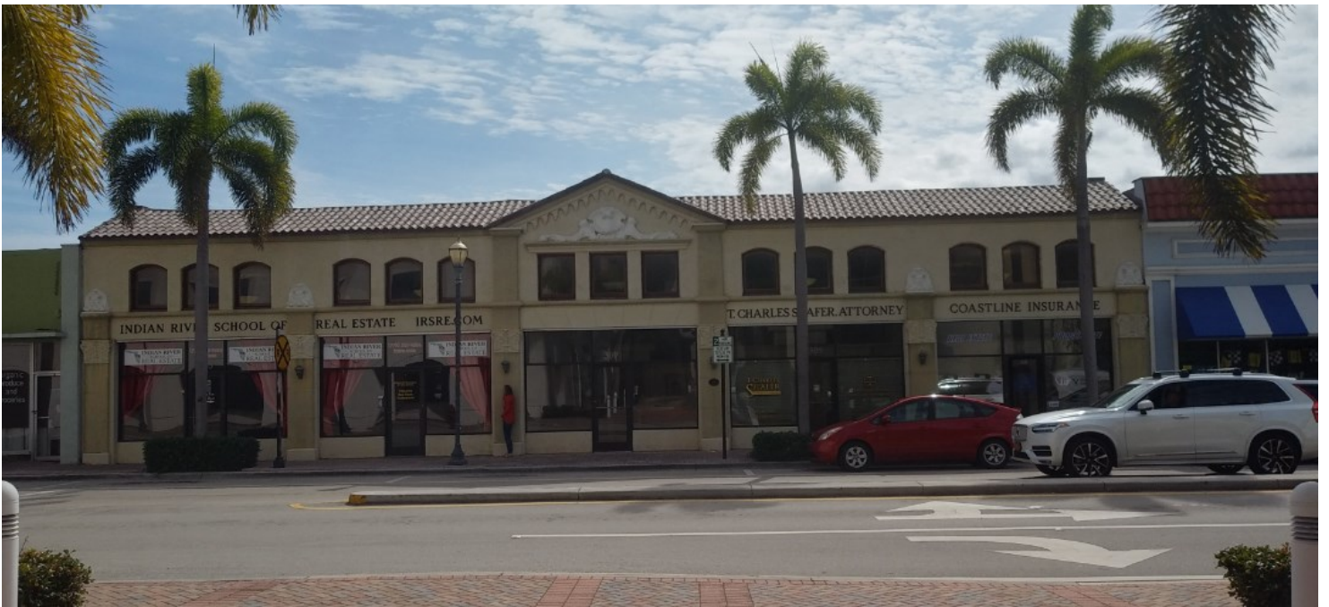
Existing front facade
