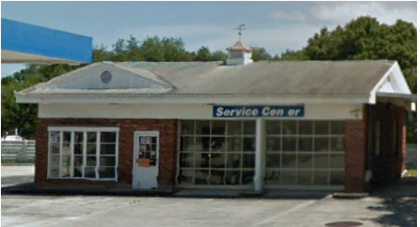
EXISTING FRONT FAÇADE
