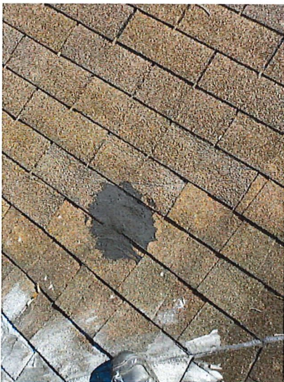
Project: 701 S 7th St Date: April 3rd, 2020, 10:43 a.m. Creator: Ray Davis
