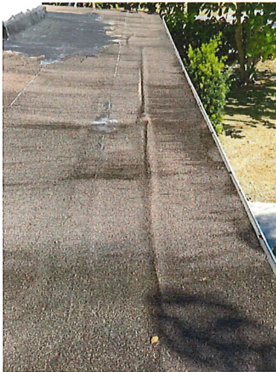
Project: 701 S 7th St Date: April 3rd, 2020, 10:41 a.m. Creator: Ray Davis
