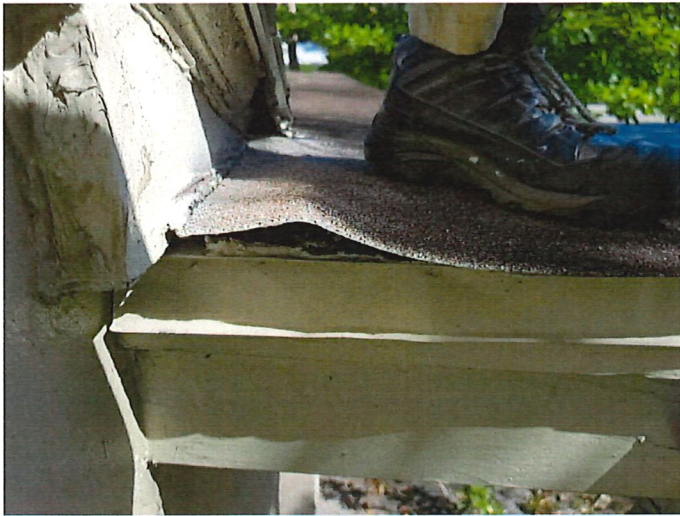
Project: 701 S 7th St Date: April 3rd, 2020, 10:40 a.m. Creator: Ray Davis
