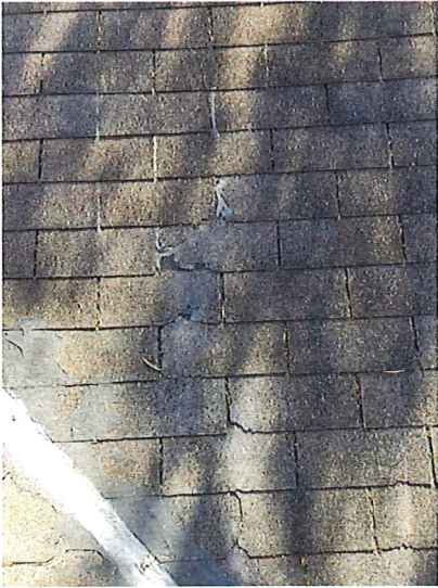
Project: 701 S 7th St Date: April 3rd, 2020, 10:39 a.m. Creator: Ray Davis
