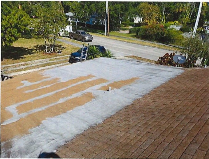
Project: 701 S 7th St Date: April 3rd, 2020, 10:43 a.m. Creator: Ray Davis
