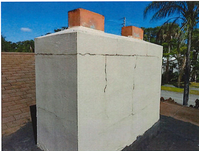
Project: 701 S 7th St Date: April 3rd, 2020, 10:42 a.m. Creator: Ray Davis
