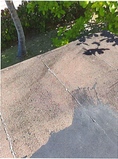
Project: 701 S 7th St Date: April 3rd, 2020, 10:42 a.m. Creator: Ray Davis
