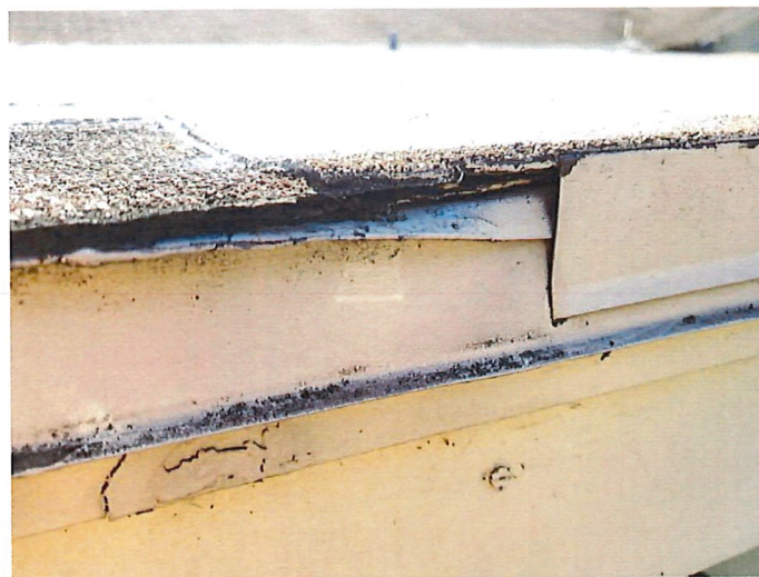
Project: 701 S 7th St Date: April 3rd, 2020, 10:36 a.m. Creator: Ray Davis
