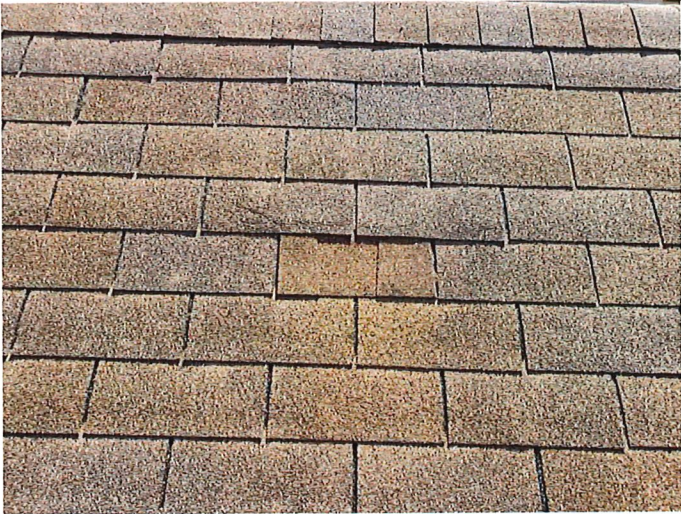
Project: 701 S 7th St Date: April 3rd, 2020, 10:37 a.m. Creator: Ray Davis
