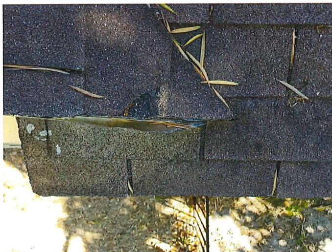
Project: 701 S 7th St Date: April 3rd, 2020, 10:40 a.m. Creator: Ray Davis
