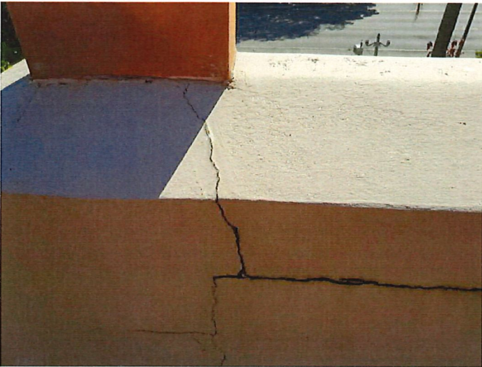
Project: 701 S 7th St Date: April 3rd, 2020, 10:41 a.m. Creator: Ray Davis
