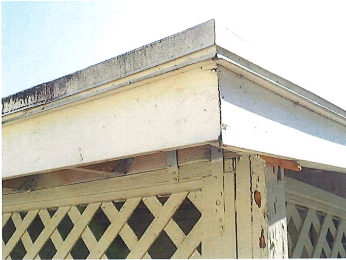
Project: 701 S 7th St Date: April 3rd, 2020, 10:35 a.m. Creator: Ray Davis
