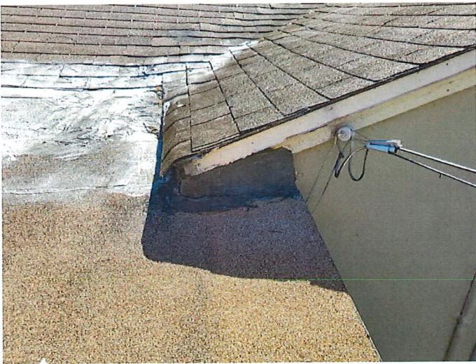
Project: 701 S 7th St Date: April 3rd, 2020, 10:38 a.m. Creator: Ray Davis
