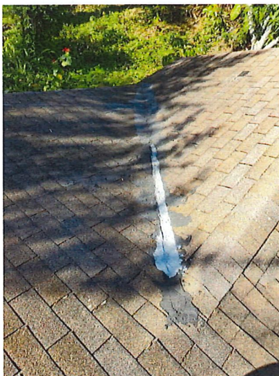
Project: 701 S 7th St Date: April 3rd, 2020, 10:38 a.m. Creator: Ray Davis
