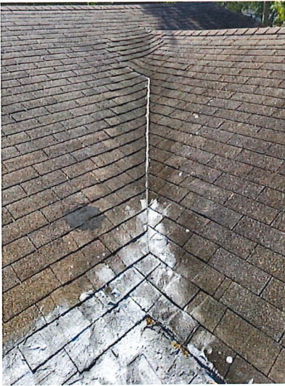
Project: 701 S 7th St Date: April 3rd, 2020, 10:37 a.m. Creator: Ray Davis
