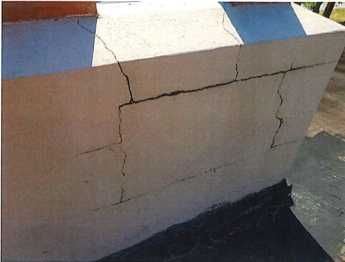
Project: 701 S 7th St Date: April 3rd, 2020, 10:41 a.m. Creator: Ray Davis
