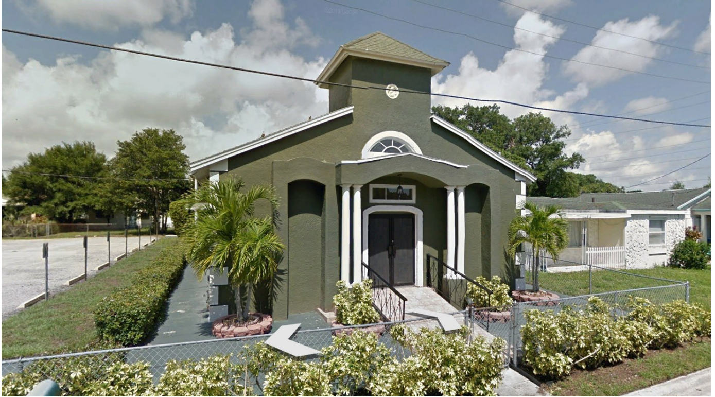
Church building with existing fence
