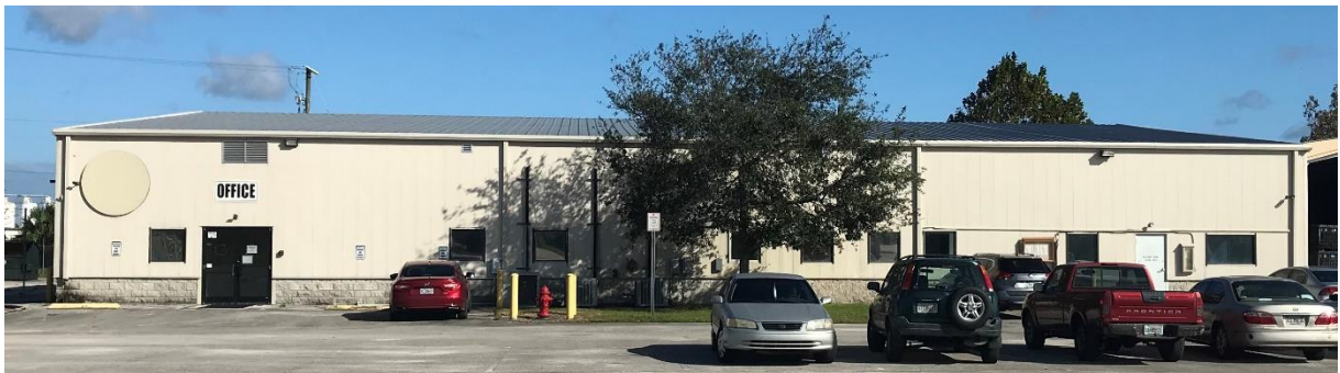
Building 2 – Large warehouse (temporary structures are being removed)
