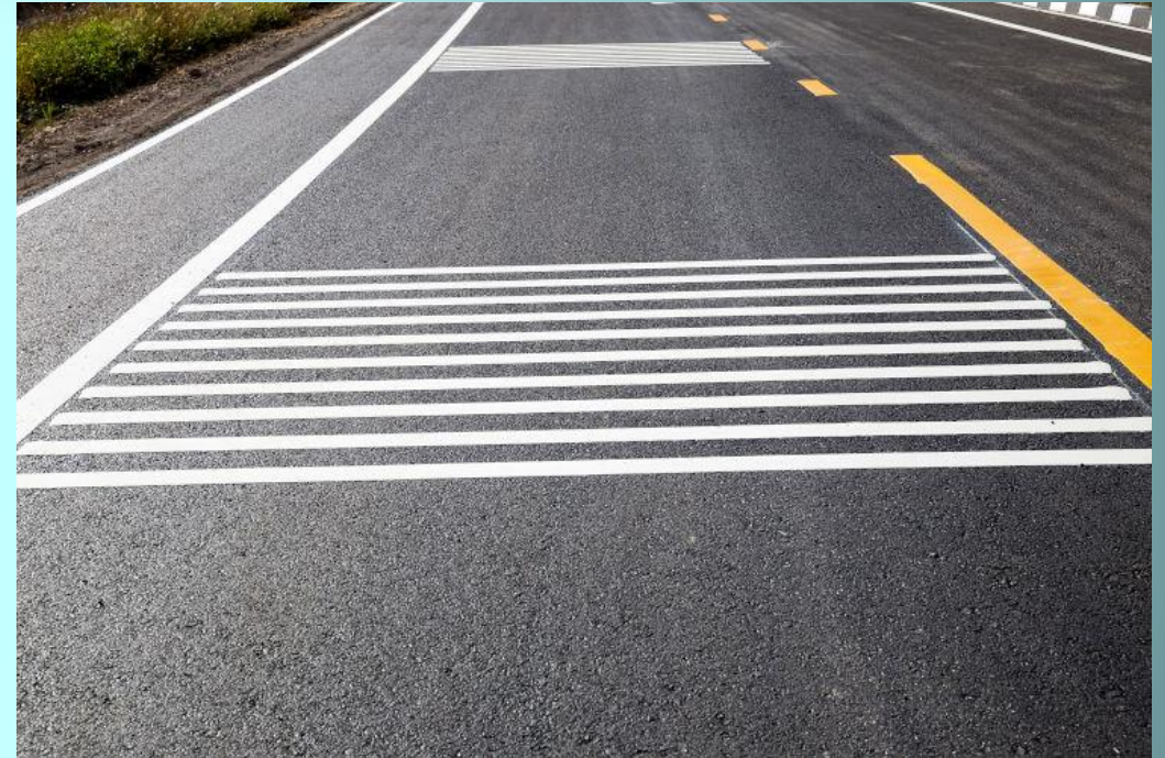
Transverse Pavement Markings At Stop Sign Approaches
