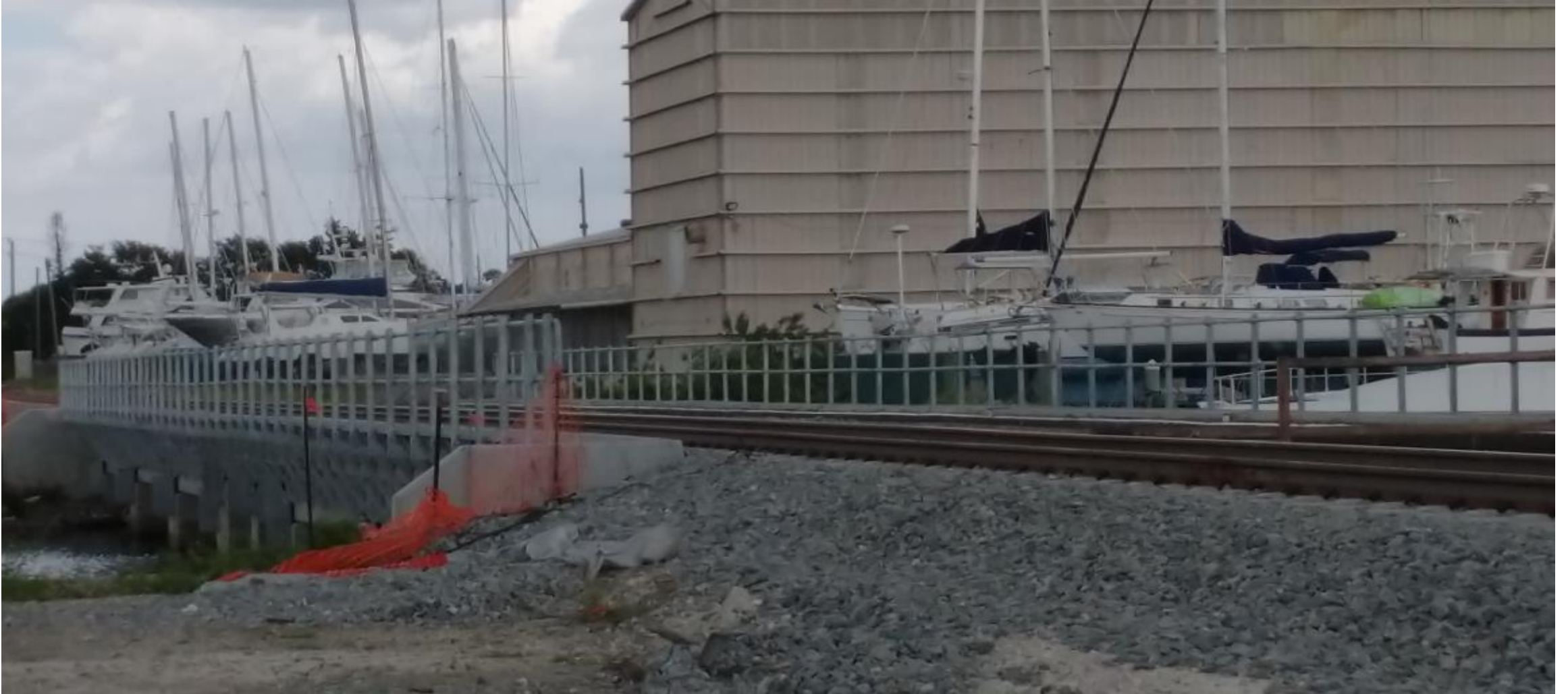
North Old Dixie Hwy - Railroad Bridge
