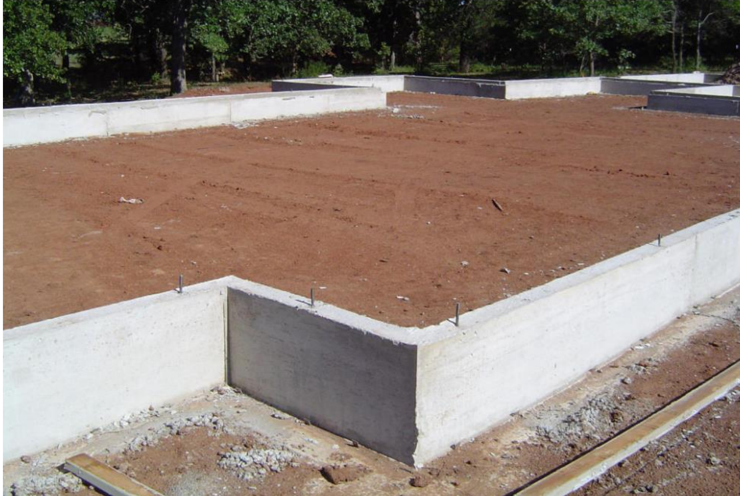
Stemwall Construction
