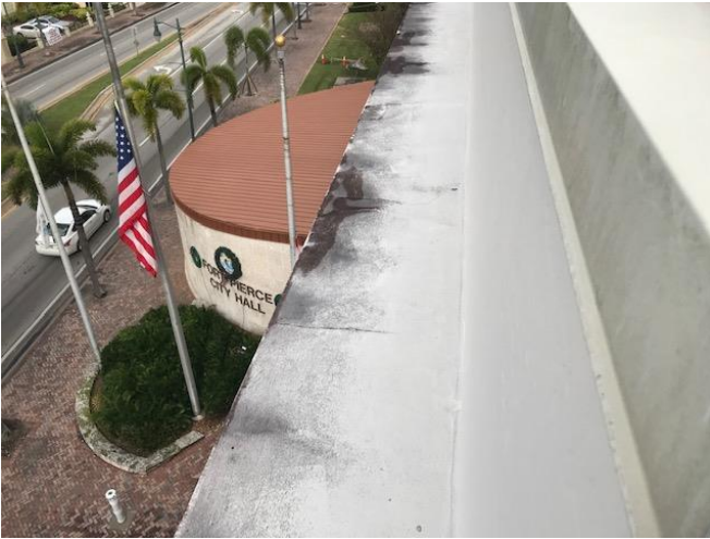
Top horizontal band of box out to receive Sto cementitious waterproofing membrane
