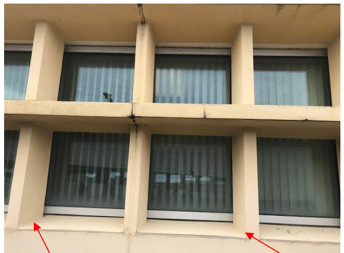
Caulking of 90 degree angles
