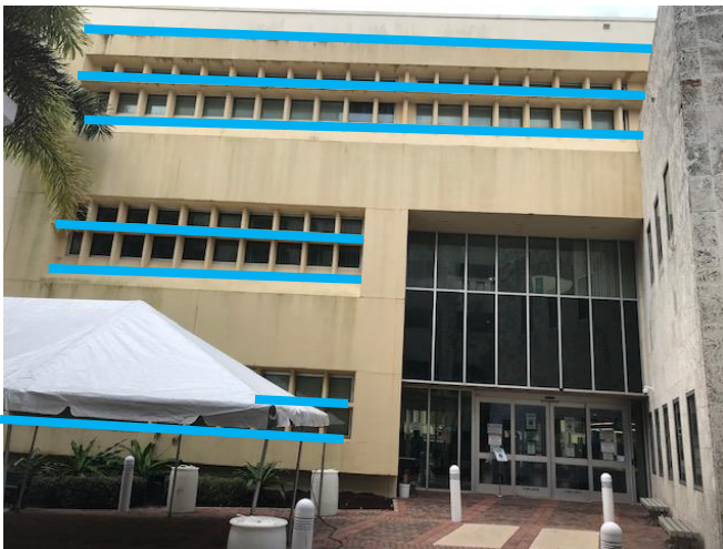
Seven ledges total (end to end) for Sto installation (marked in blue)
