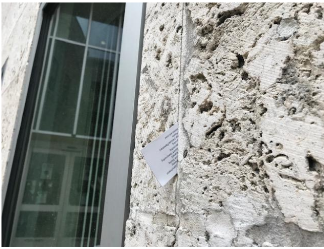
Tuck pointing and penetrating sealer
