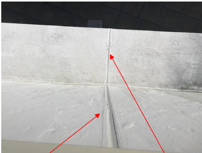
Reveal joint caulking Vertical reveal joint – Top of box out
