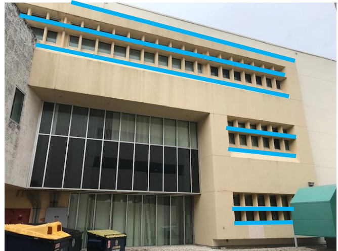
Seven ledges total (end to end) for Sto installation (marked in blue)
