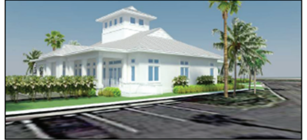
LOOKING NORTH EAST
