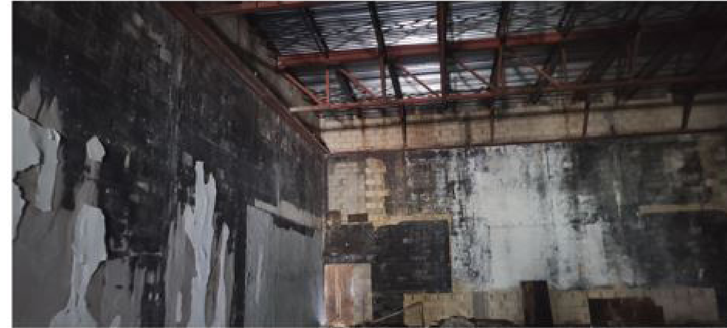
Existing Wall Conditions With Roof Structure
