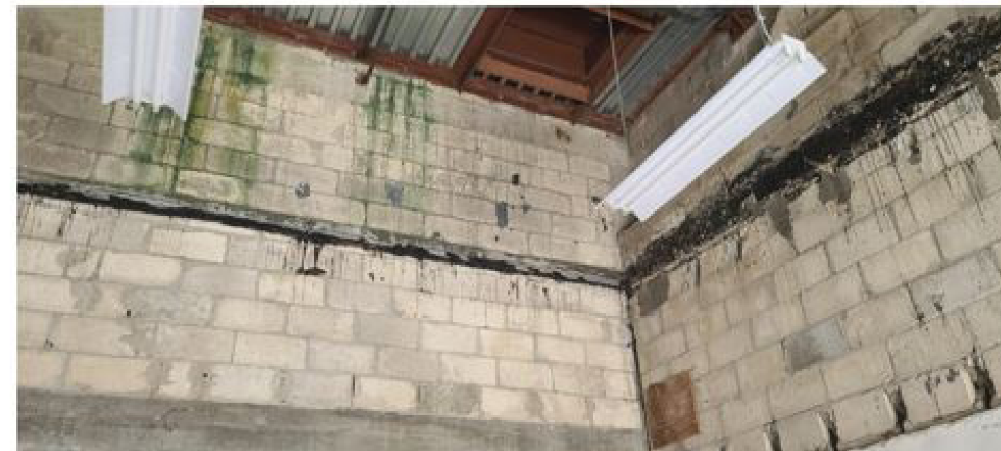
Existing Lobby Wall Condition
