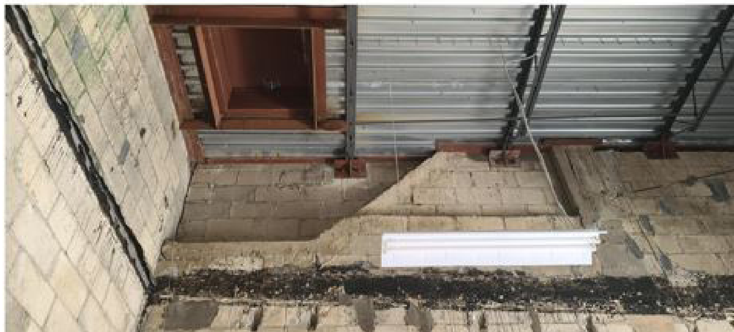
Existing Lobby Roof Structure (Looking at the Gorter)
