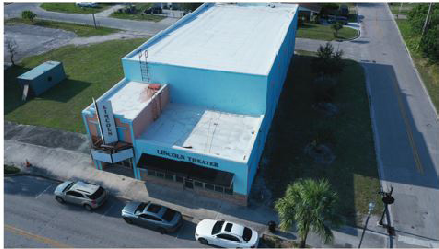
Existing South Facade (South Aerial)
