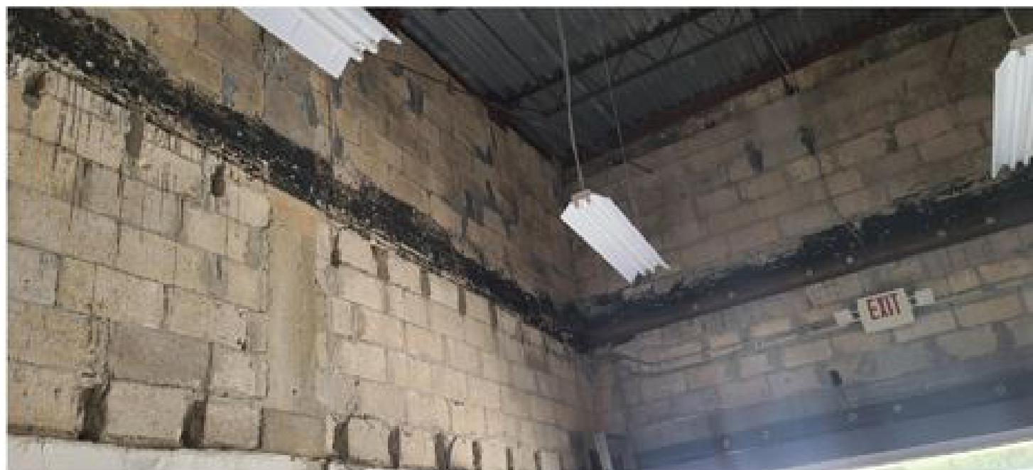
Existing Wall Conditions
