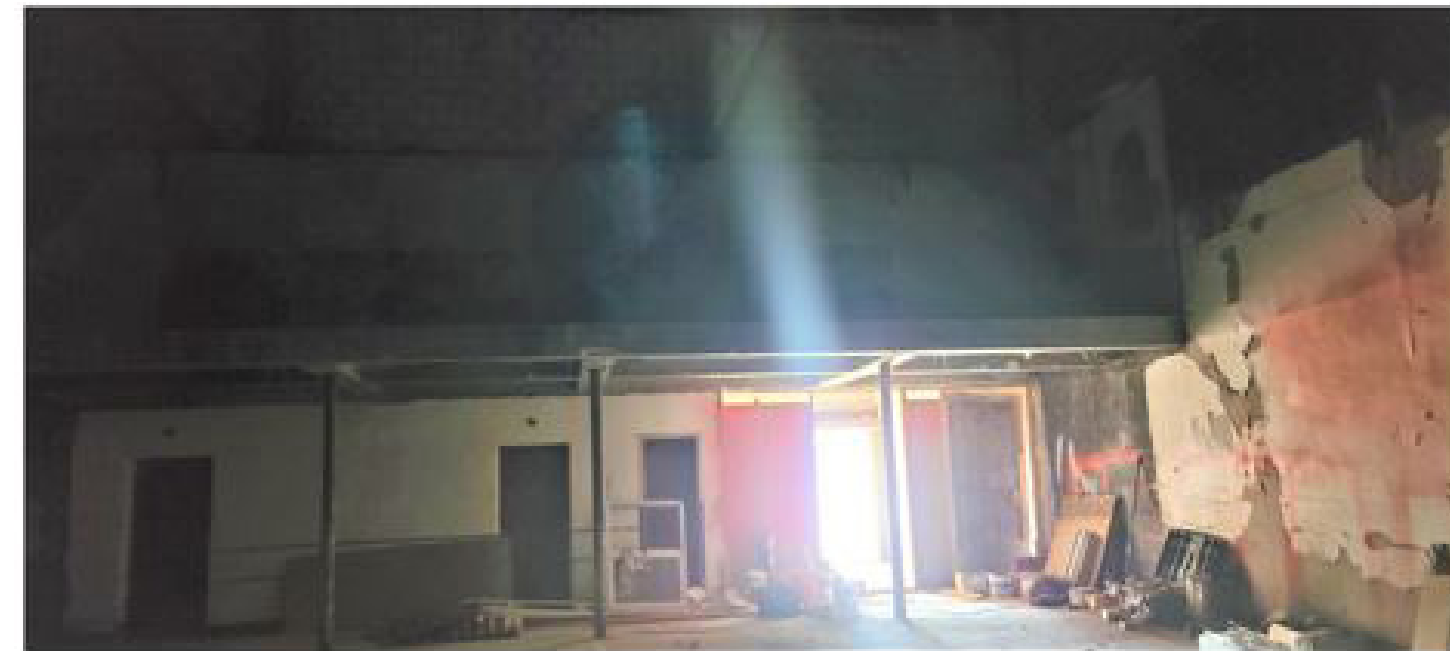
Existing Column Structure with Views of Main Entrance and Bathrooms
