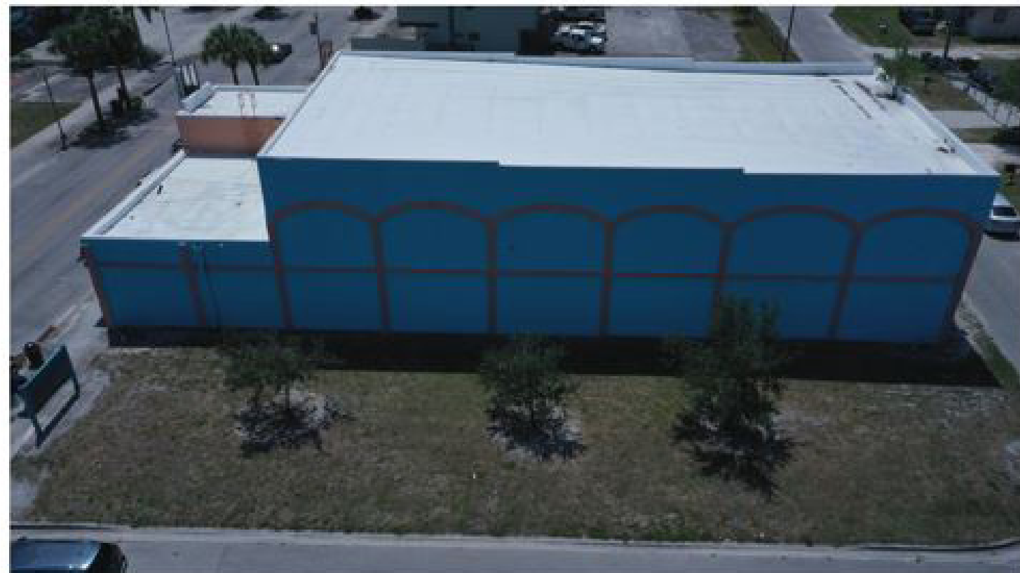
Existing Facade (East)
