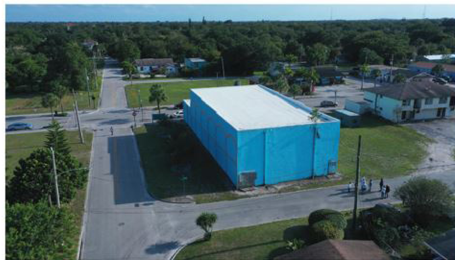
Existing North Facade (Rear)
