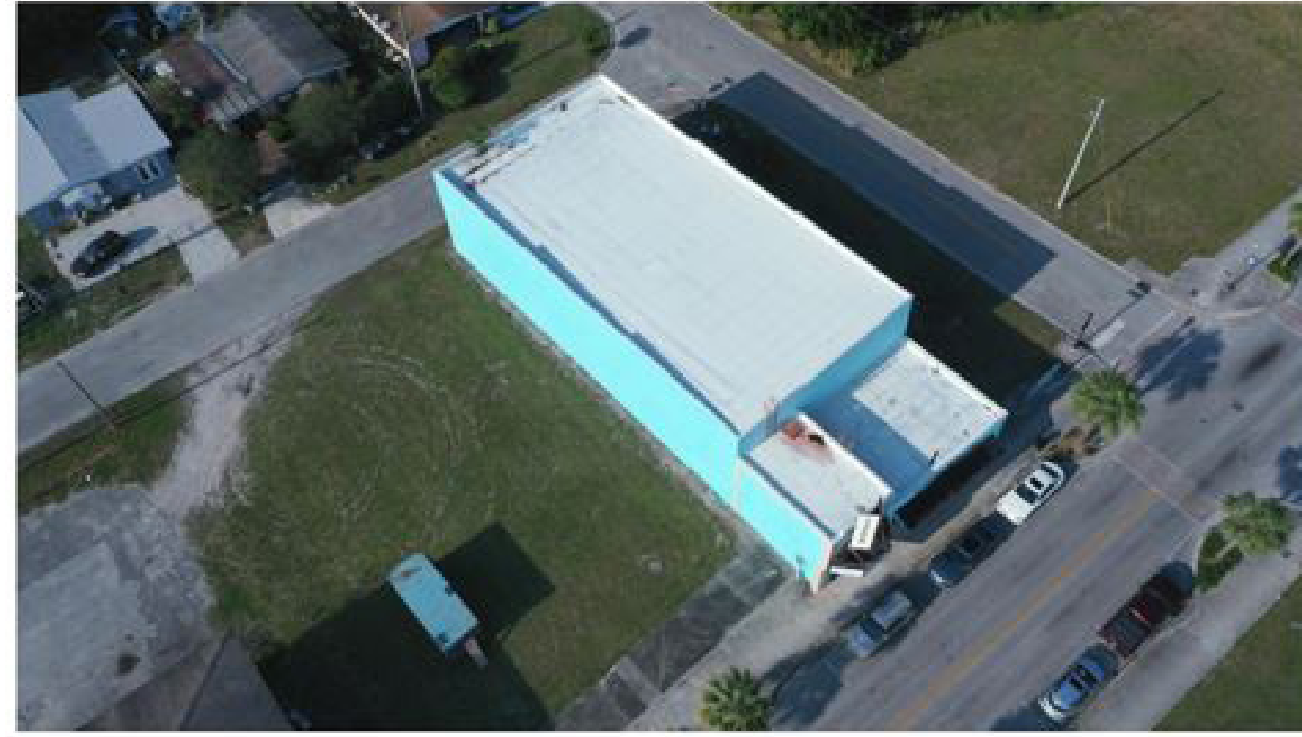
Site/Building Aerial (North East)
