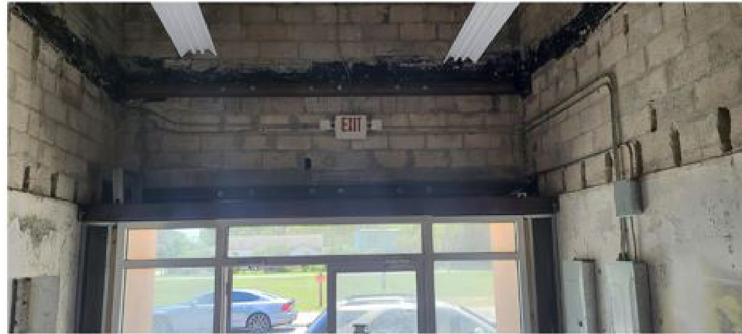
Existing Lobby Storefront
