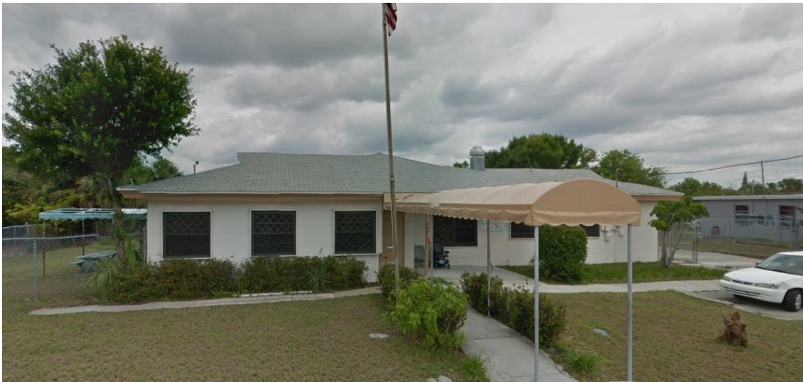
FRONT FAÇADE OF THE SUBJECT BUILDING
