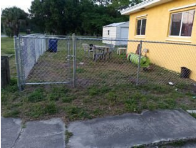
4 foot chain link fence
