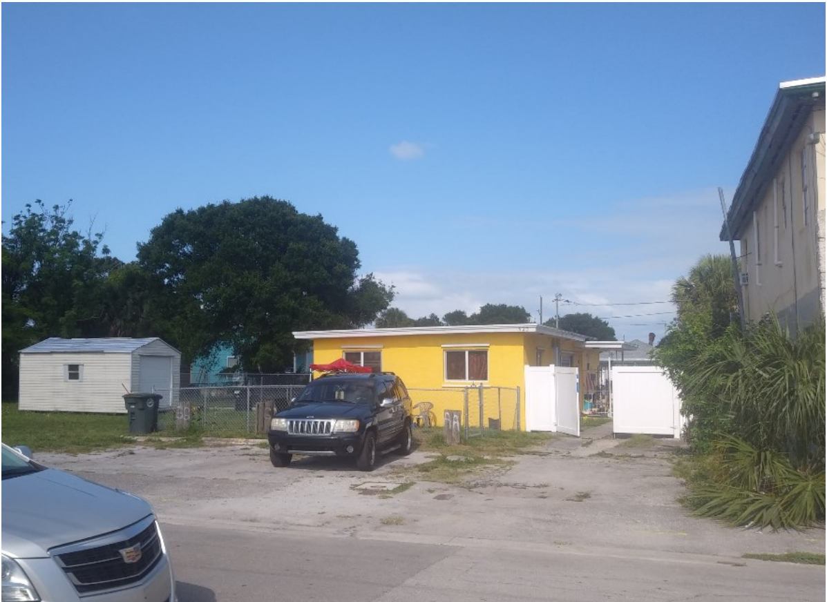
Front yard view/chain link and PVC fences
