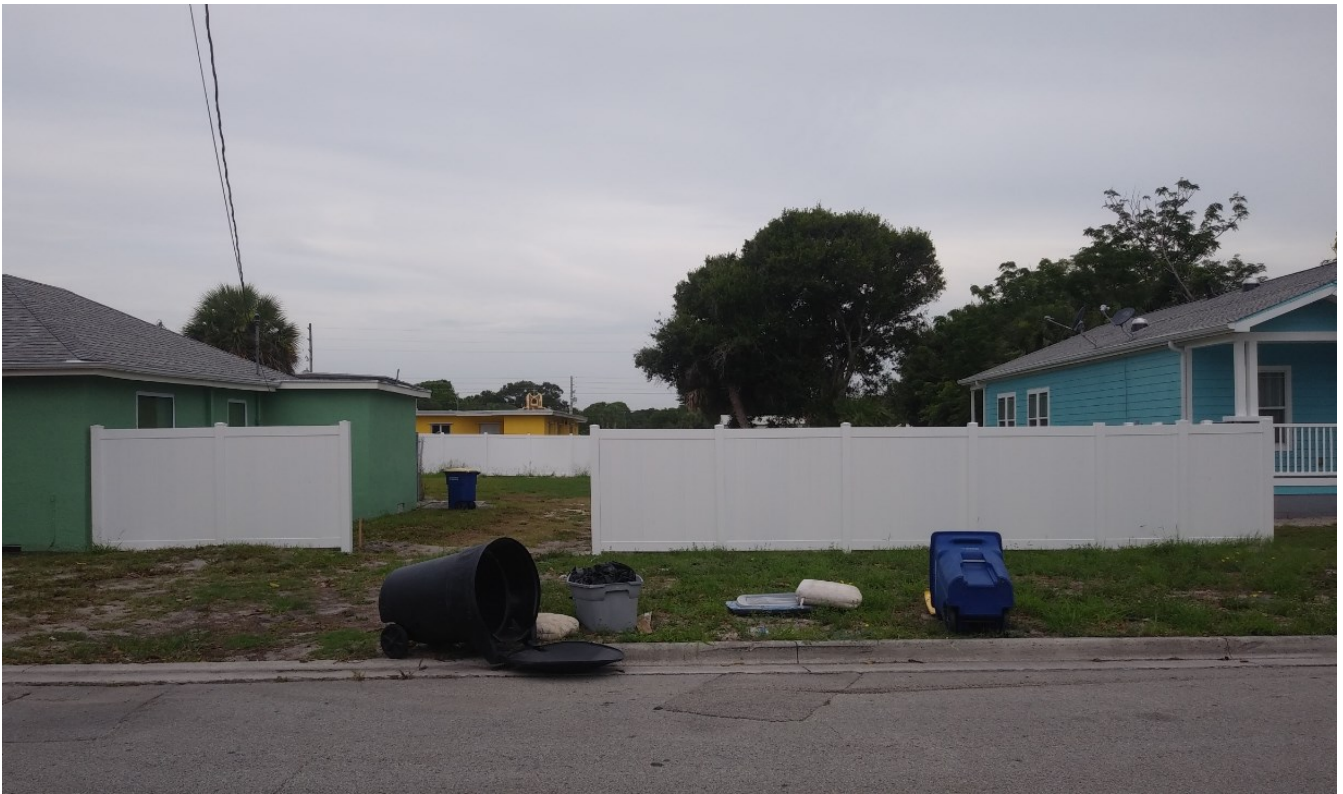
View of the 6 foot PVC fence within front yard
