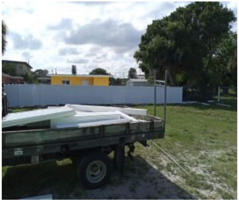
6 foot PVC fence on the rear property line
