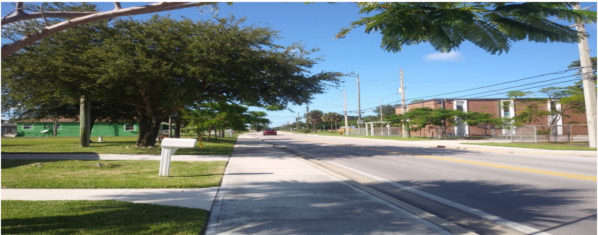
13th Street view looking north
