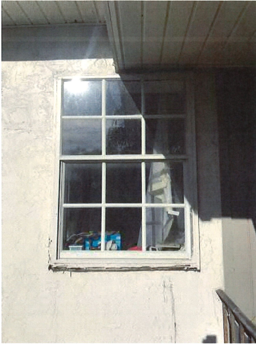
Kitchen - Floor 1 Line Item: 4
