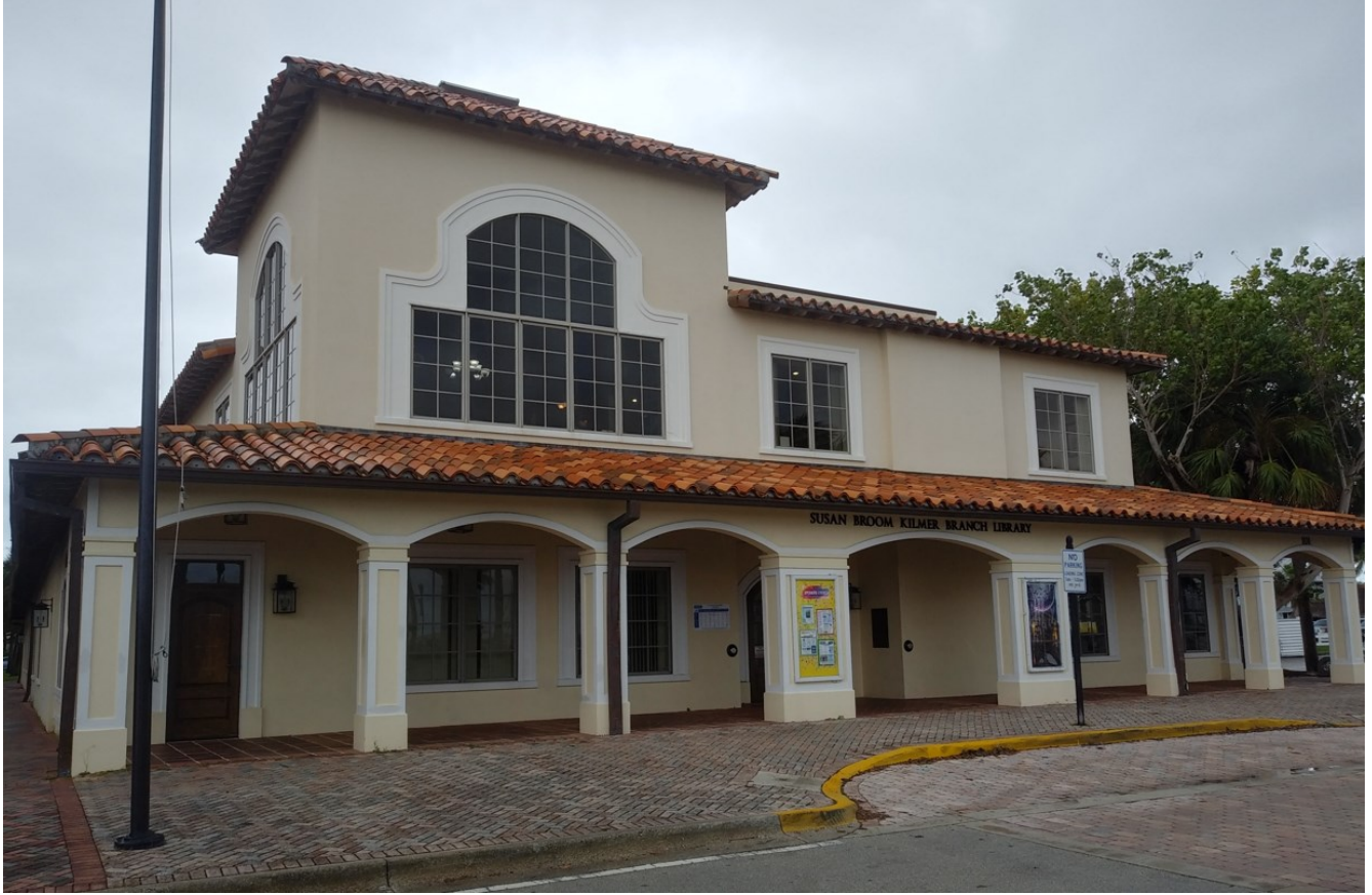
LIBRARY — EAST/FRONT FACADE
