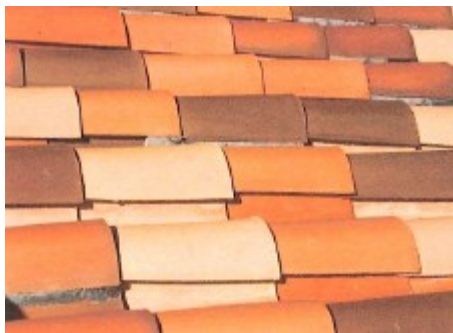
CRACKED AND SHIFTED TILES AND LOOSE MORTAR NOTED THROUGHOUT THE FIELD OF THE ROOF.
