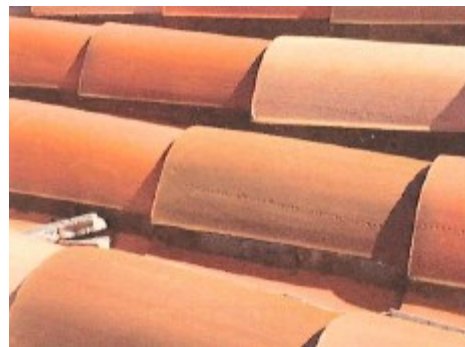
CRACKED AND SHIFTED TILES AND LOOSE MORTAR NOTED THROUGHOUT THE FIELD OF THE ROOF.
