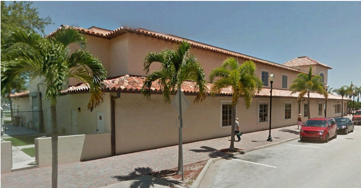
LIBRARY — SOUTH/SIDE FAÇADE
