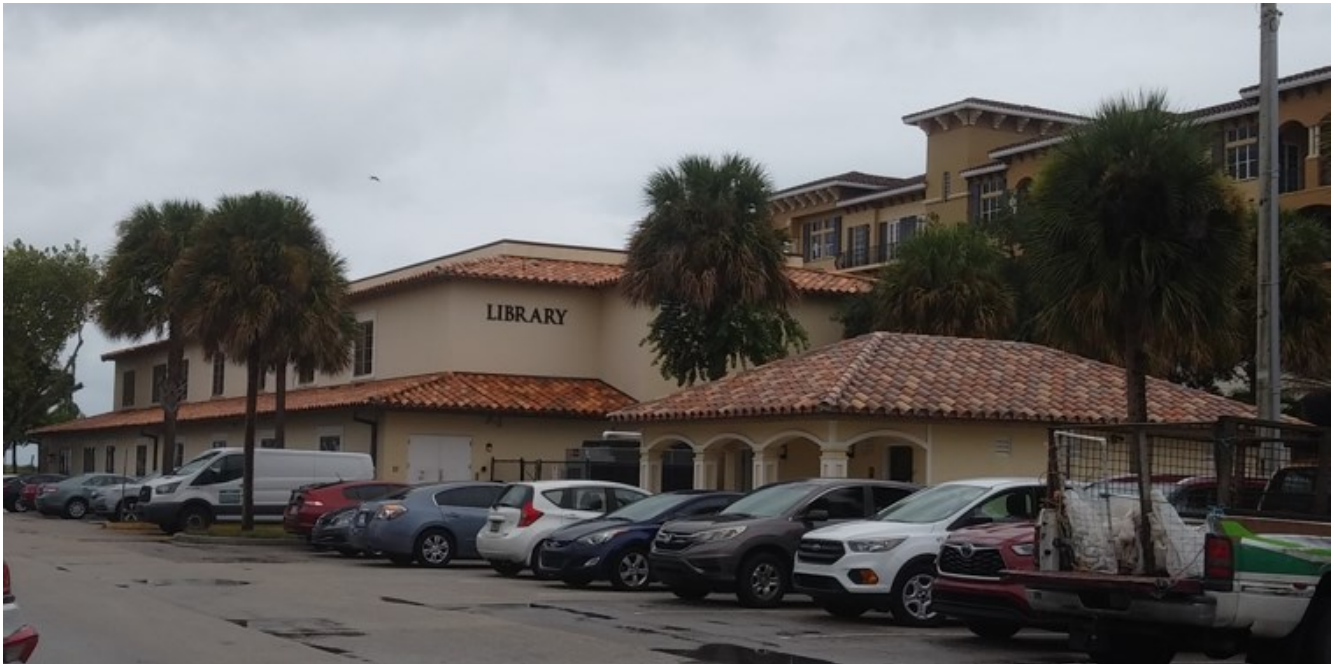
LIBRARY & RESTROOMS — NORTH/SIDE FACADE
