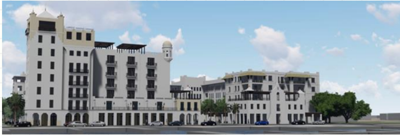
EAST ELEVATION – MAY 24, 2021
