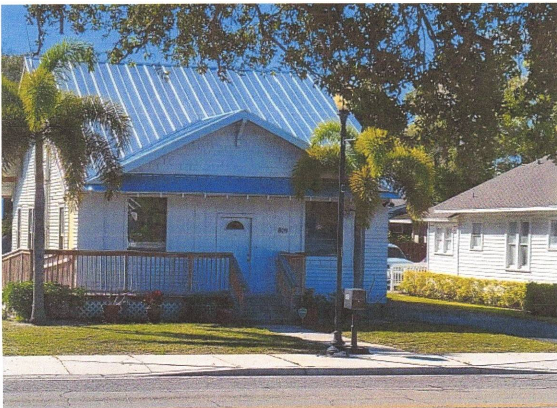
DELAWARE AVENUE FAÇADE
