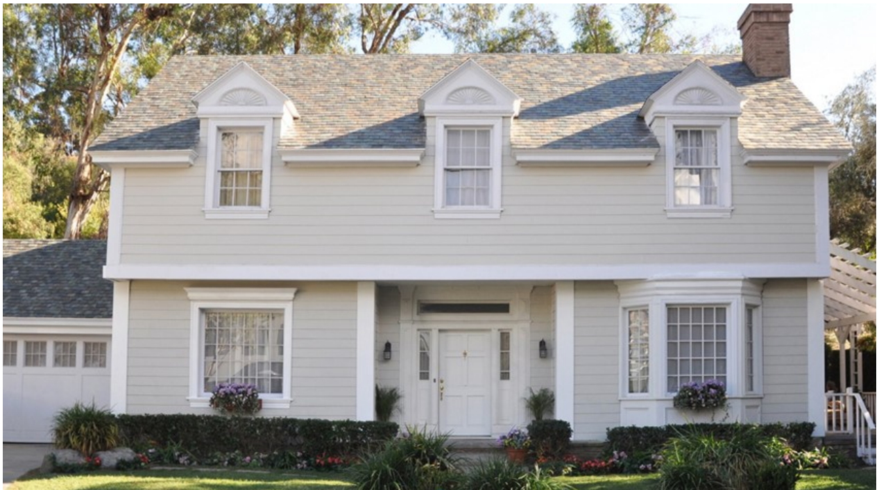
HOMES WITH A NEWLY INSTALLED TESLA SOLAR ROOF. COURTESY TESLA
