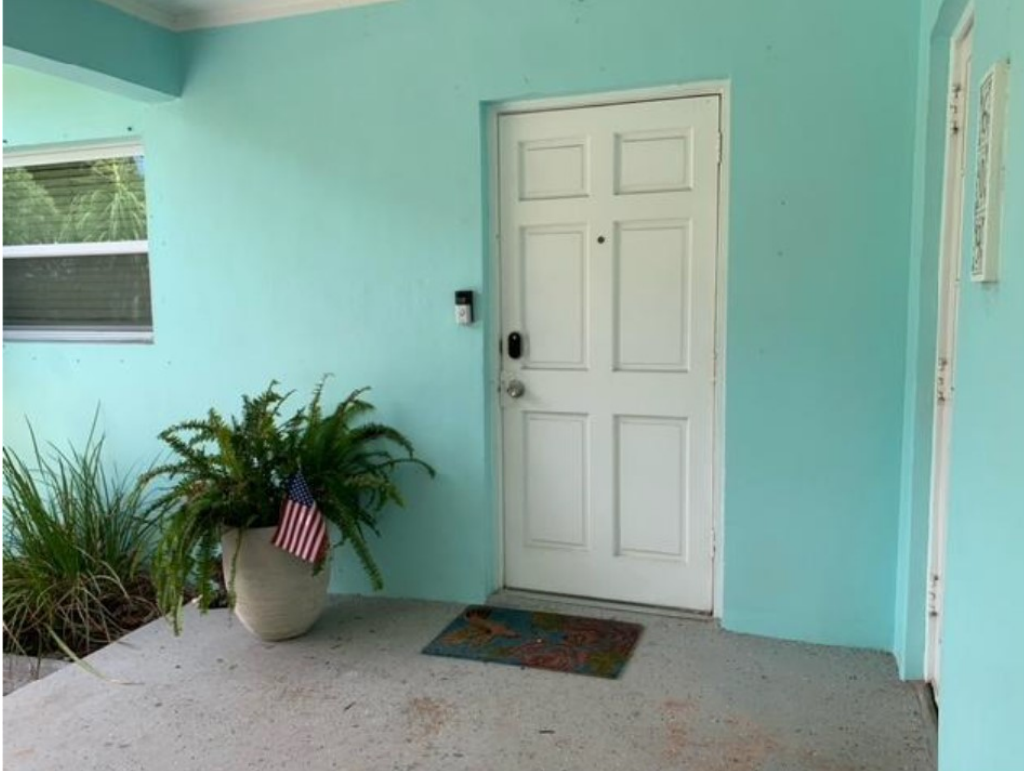
EXISTING FRONT DOOR: OPENING TO BE WIDENED AND DOOR REPLACED
