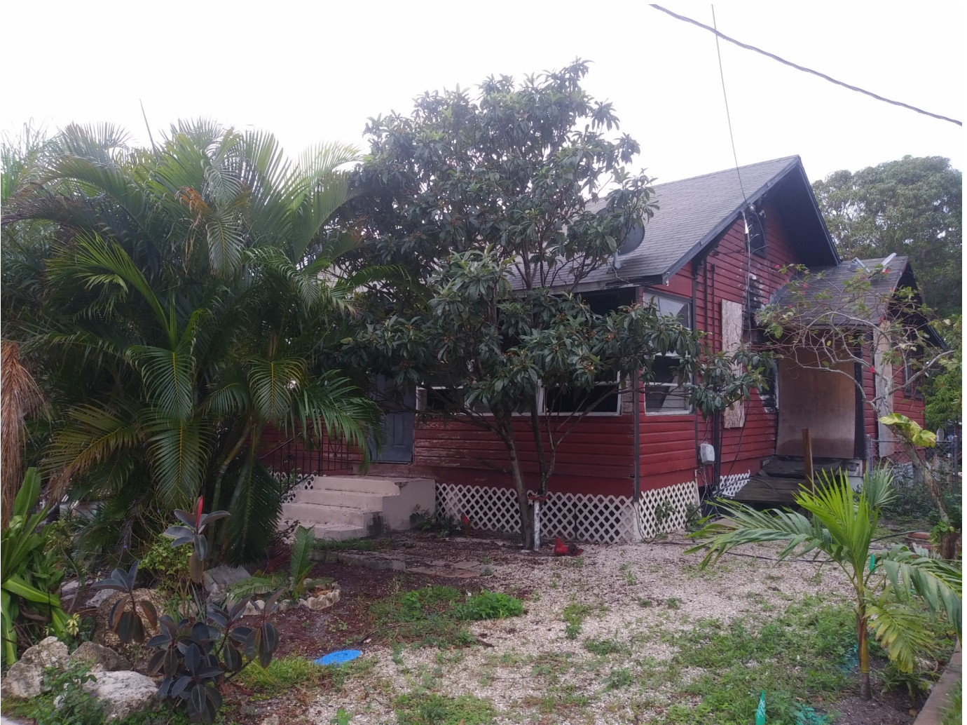
Existing structure front/side facade
