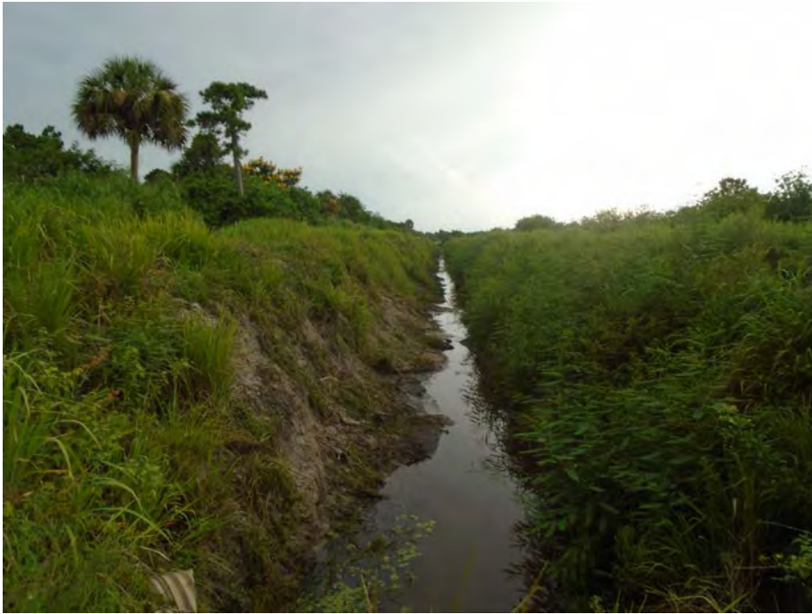
15. West View: Drainage Ditch along the North Boundary of the Subject Property
