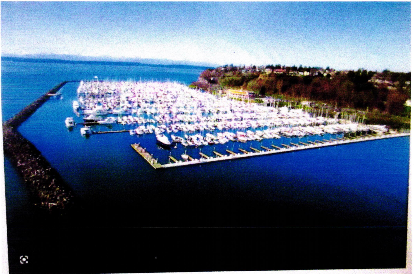
New Breakwater at Elliott Bay Marina Provides Long-Term Protection and Additional
