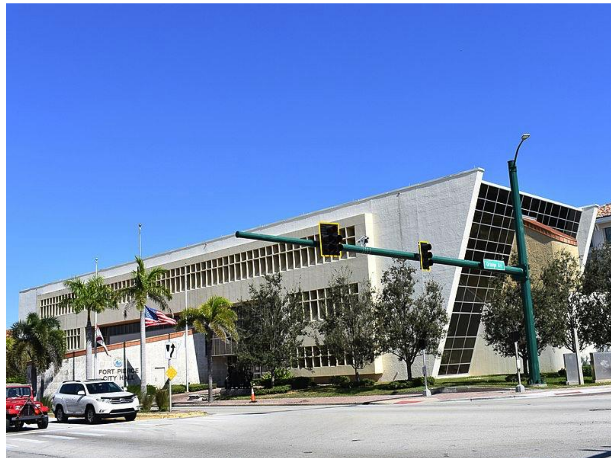
FORT PIERCE CITY HALL
