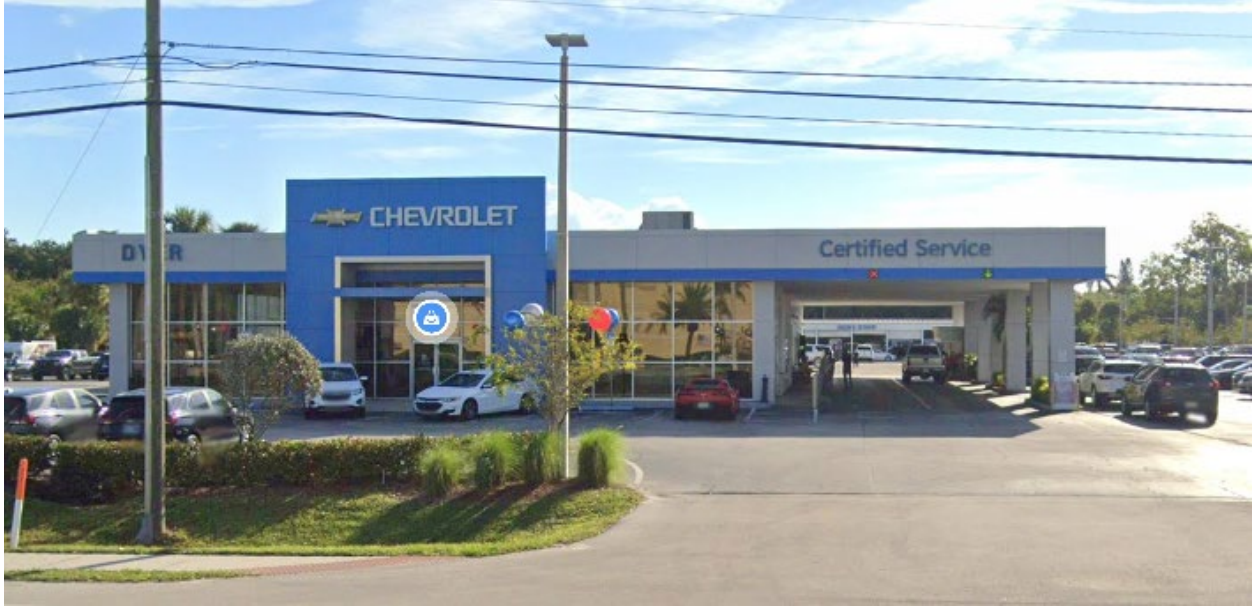
11. Adjacent Property - Dyer Chevrolet – Facing East - (ex. East side of US1, South of subject parcel)
