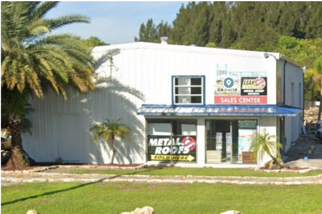
6. Leak Busters Roof Repair – Looking West – (ex. West side of US1, West of subject parcel)
