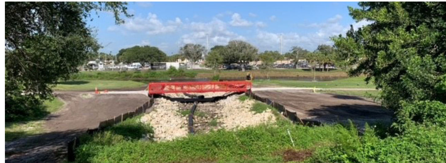
Pedestrian Bridge and Canal Stabilization
