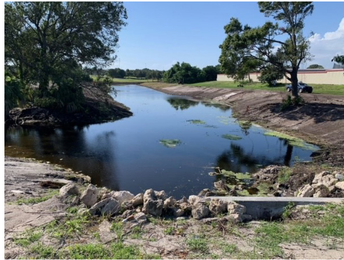
Bioswale Final Grading
