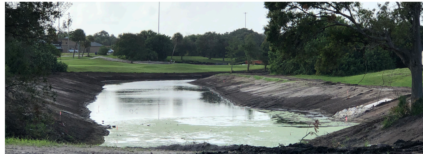
Bioswale Grading
