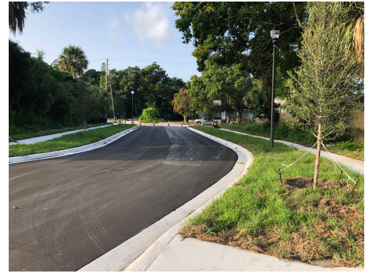
Looking South at Avenue B Roadway Connection
