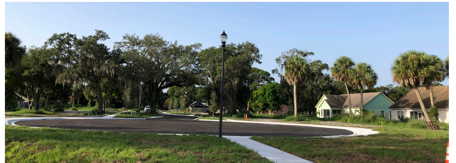
Means Court Cul-de-Sac and Sidewalk Connection to Moore's Creek Linear Park
