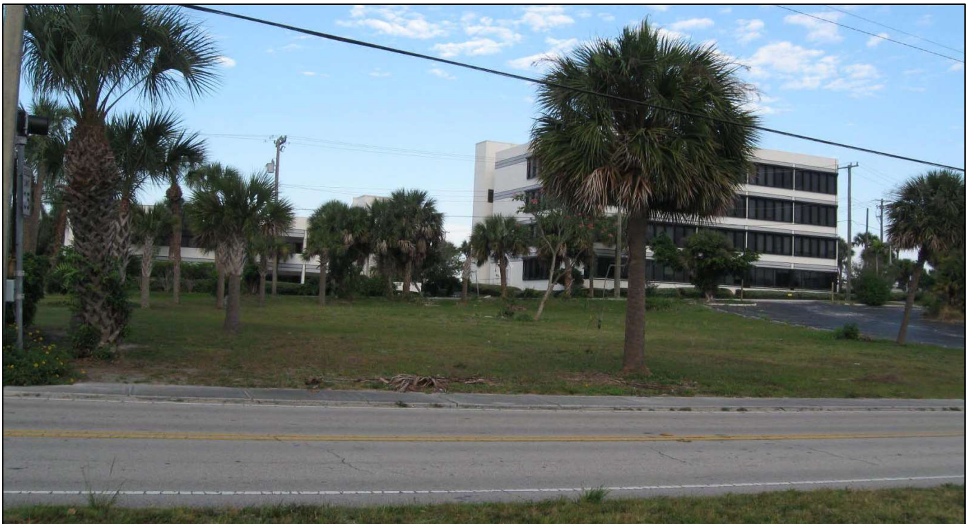
Photo looking at vacant parcel with parking area at 401 S. Indian River Drive.
