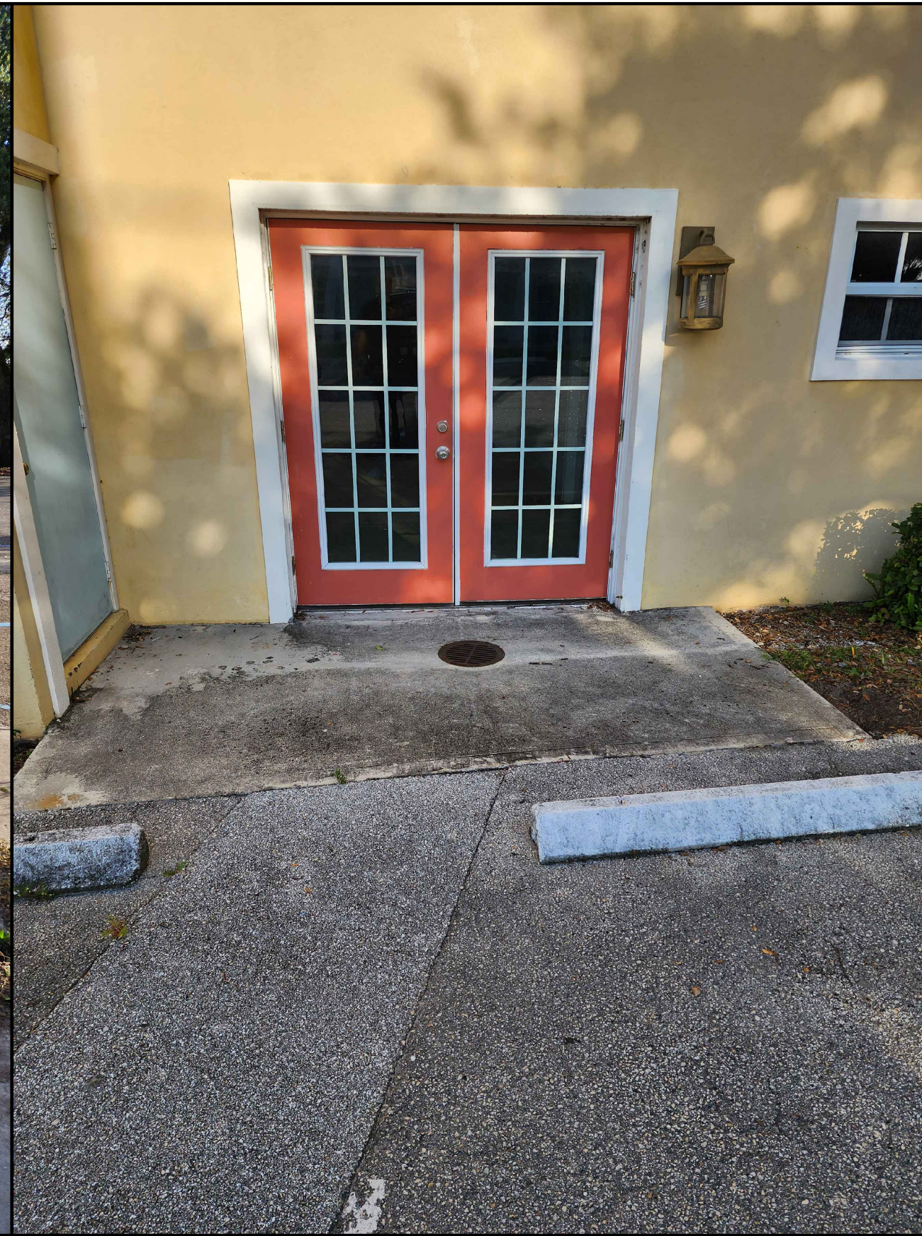
EXISTING DOUBLE DOOR MAIN ENTRY
