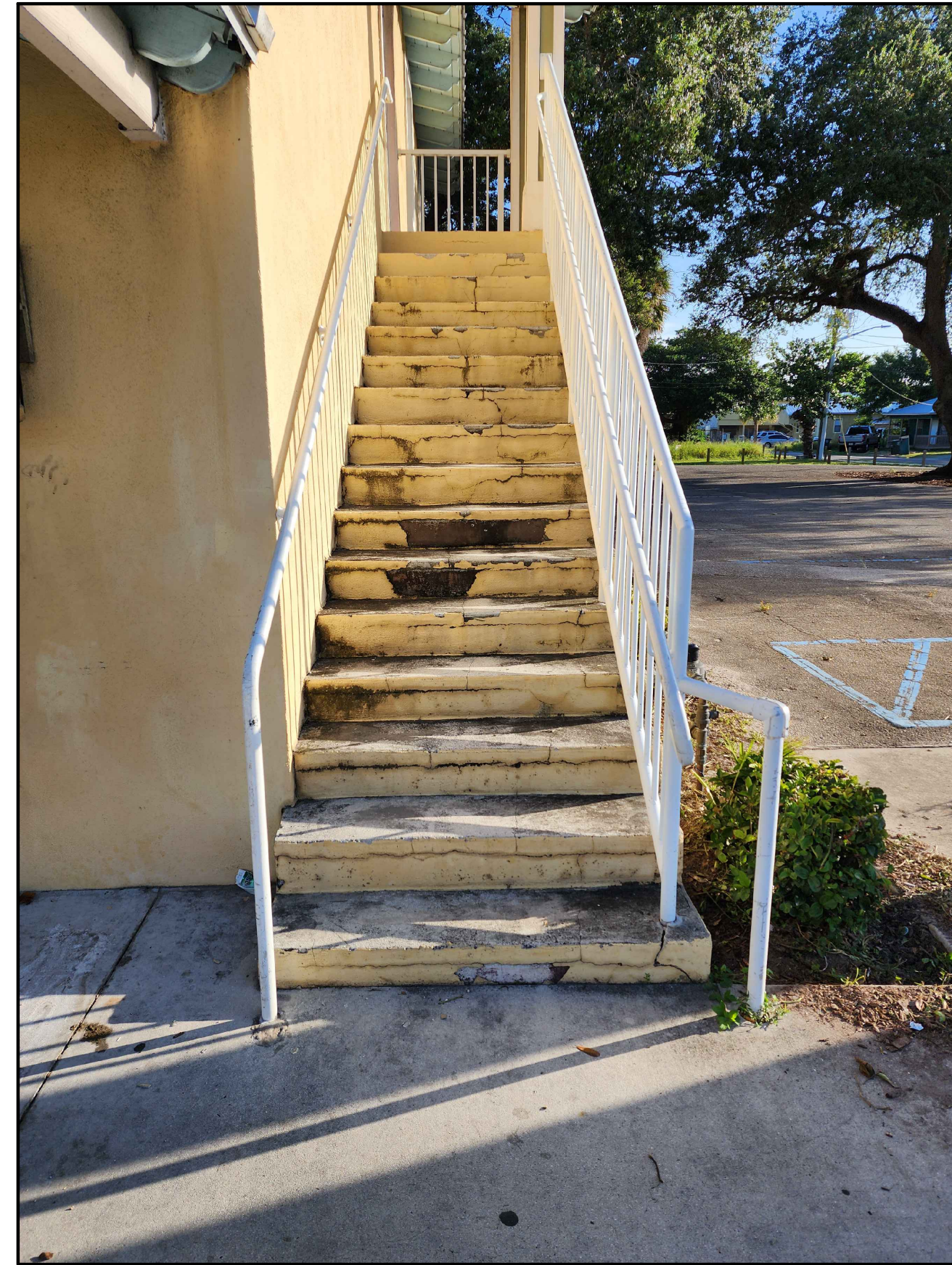
EXISTING EAST STAIR
