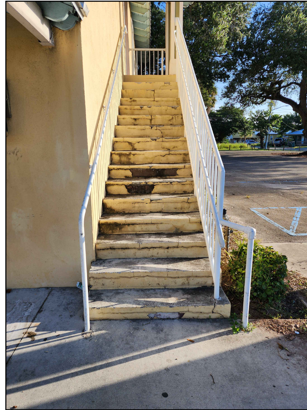
EXISTING EAST STAIR
