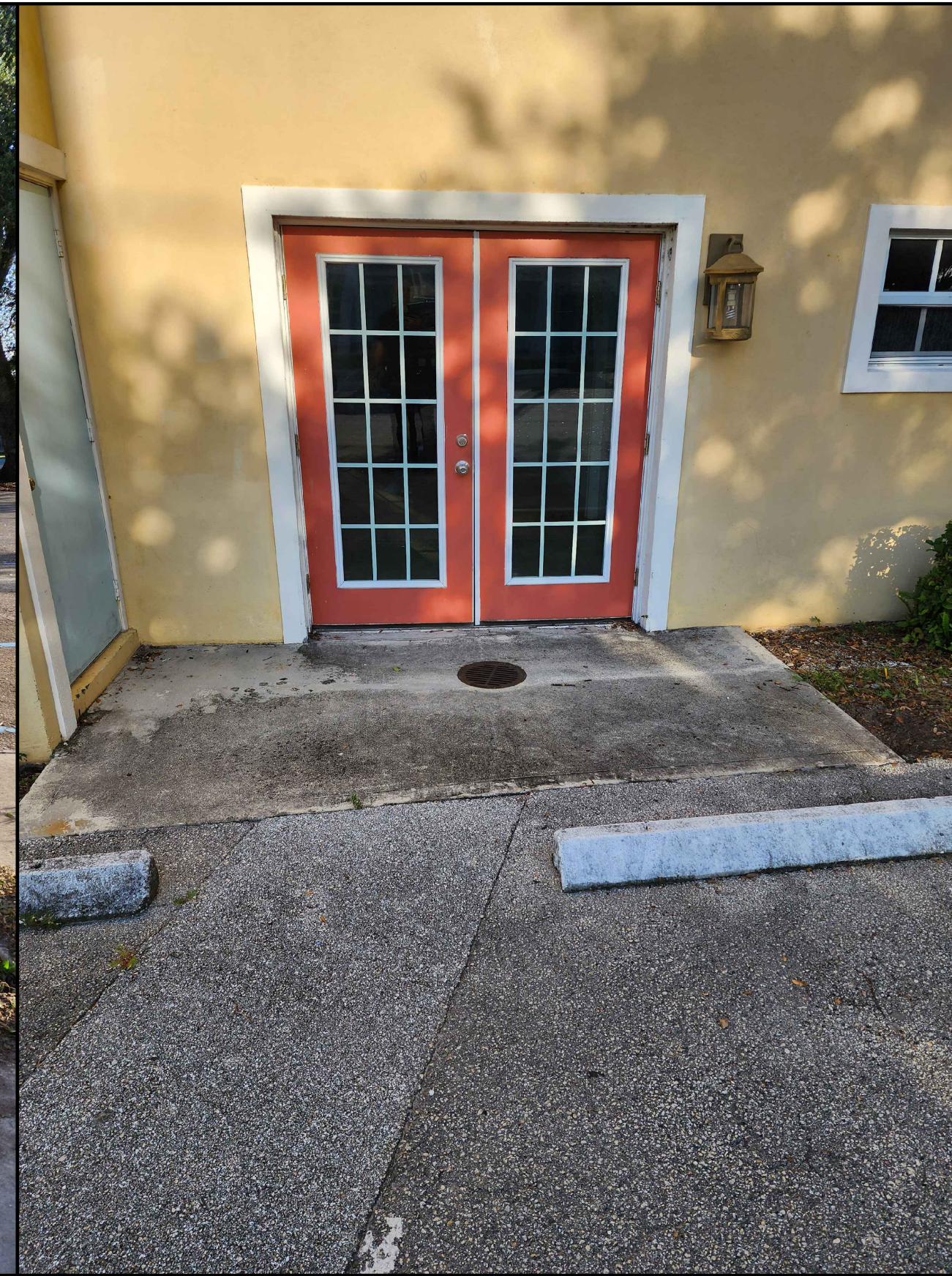
EXISTING DOUBLE DOOR MAIN ENTRY
