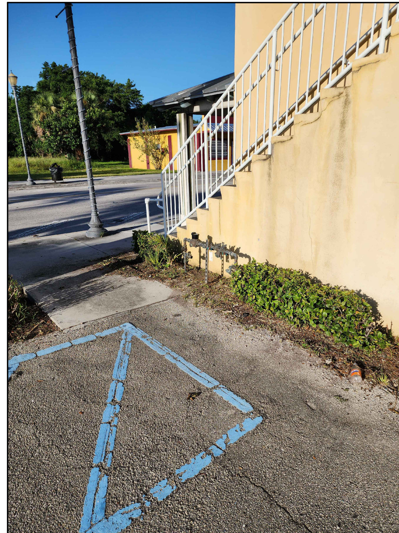
EXISTING EAST CORNER OF BUILDING LOOKING SW
