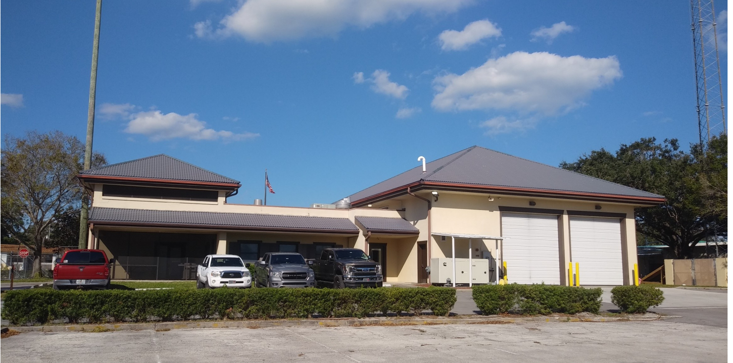
SOUTH REAR FACADE
