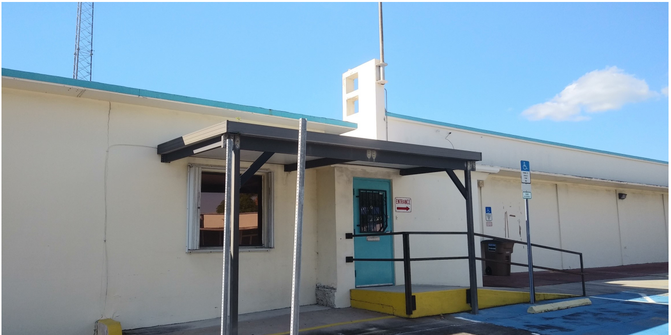
Existing structure front/east facade
