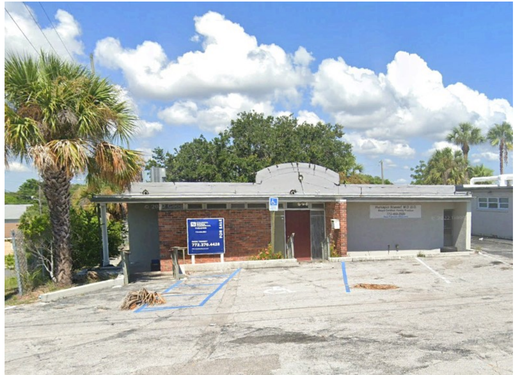
SUBJECT BUILDING - FRONT FACADE
