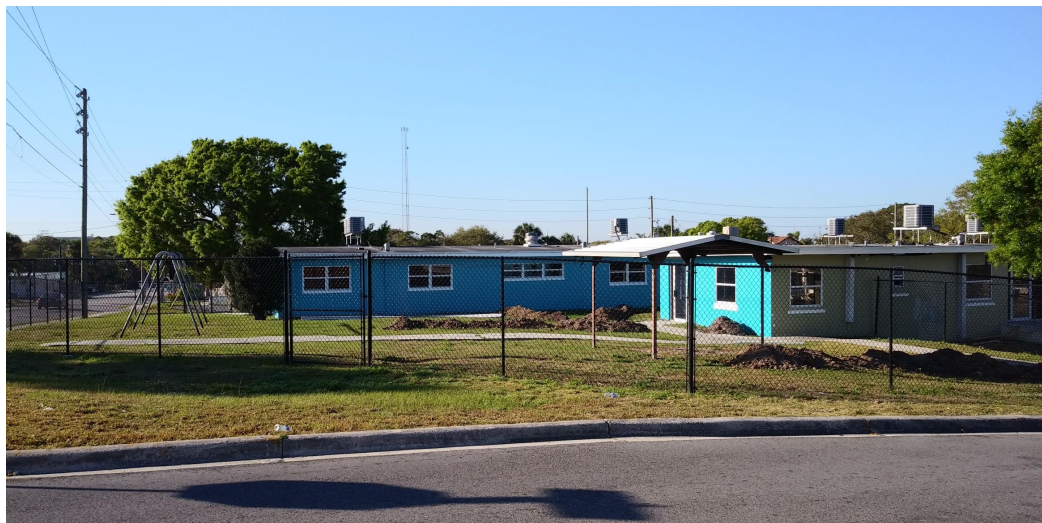
EXISTING FENCE—PROPERTY TO THE SOUTH
