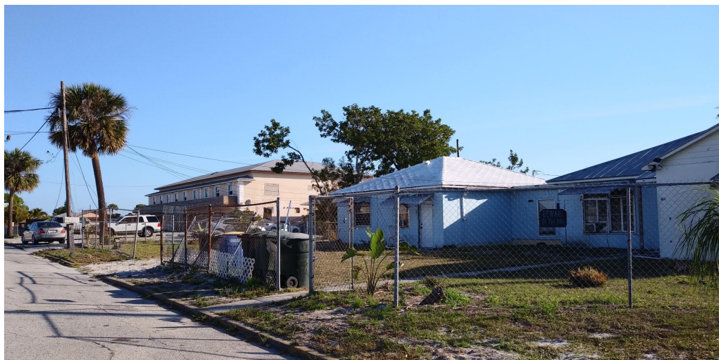
EXISTING FENCE—PROPERTY TO THE EAST
