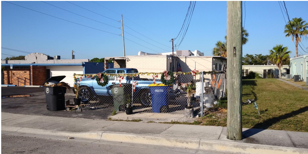
EXISTING FENCE—PROPERTY TO THE NORTH
