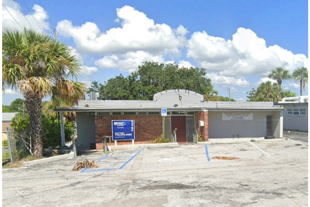
SUBJECT BUILDING - FRONT FACADE
