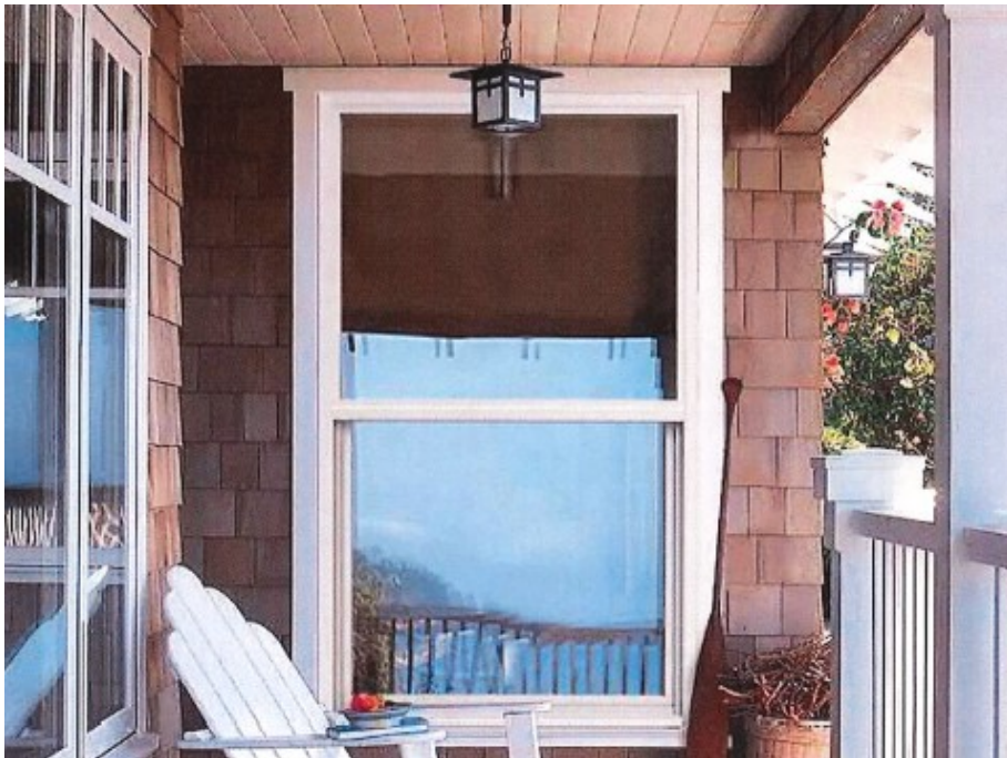
EXAMPLE OF THE WINDOWS THAT WILL BE ON THE FRONT OF HOUSE - 3050 SH IMPACT WITH SCREEN.
