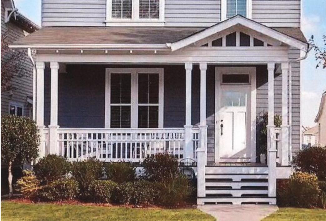
EXAMPLE OF THE DOOR THAT WILL BE ON THE FRONT OF HOUSE - 3068 SWINGING/PEDESTRIAN DOOR.
