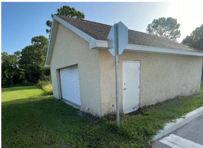
Figure 2 I.C.A. Utility Shed/Stop Sign on the northwest corner of the property
