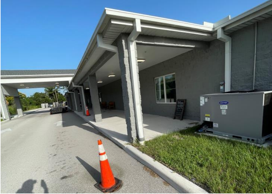
Figure 4 Northwest view of the south side of the Academy
