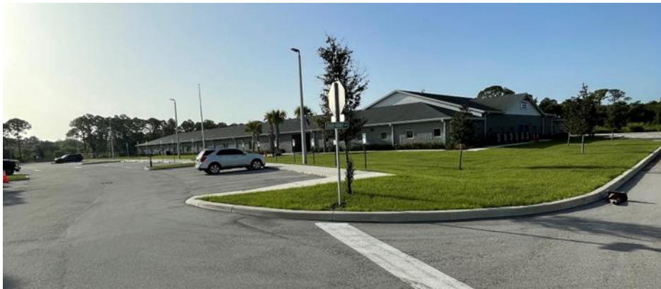
Figure 1 Northwest side view of I.C.A Main Building/Lighting Structures facing north of the building
