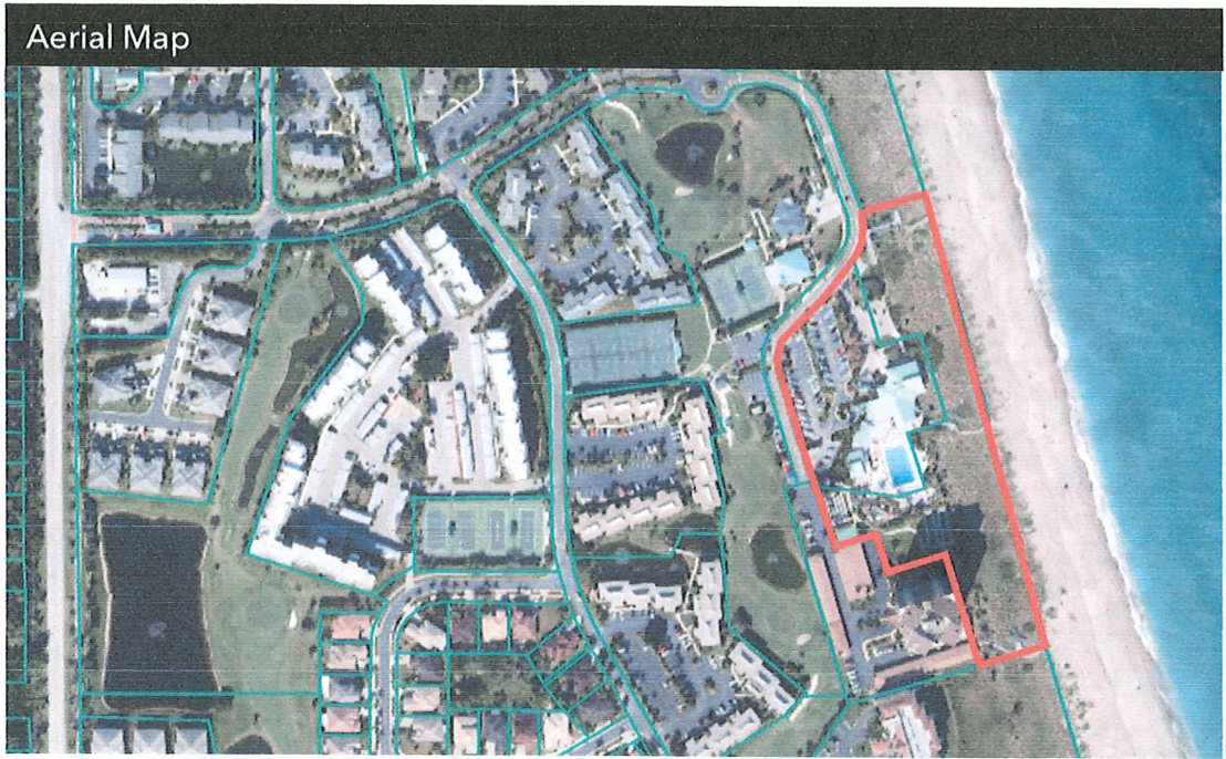
The site, outlined in red, consists of two parcels under the ownership of the Ocean Village POA, which proposes amenity improvements, and lies eastward of the CCCL.
