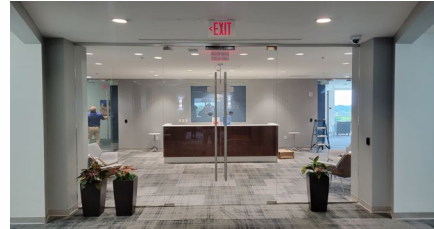
Health Trust Workforce Solutions Lobby Renovations
