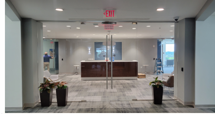
Health Trust Workforce Solutions Lobby Renovations
