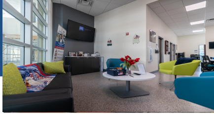
FAU Veterans Affairs Office Renovations
