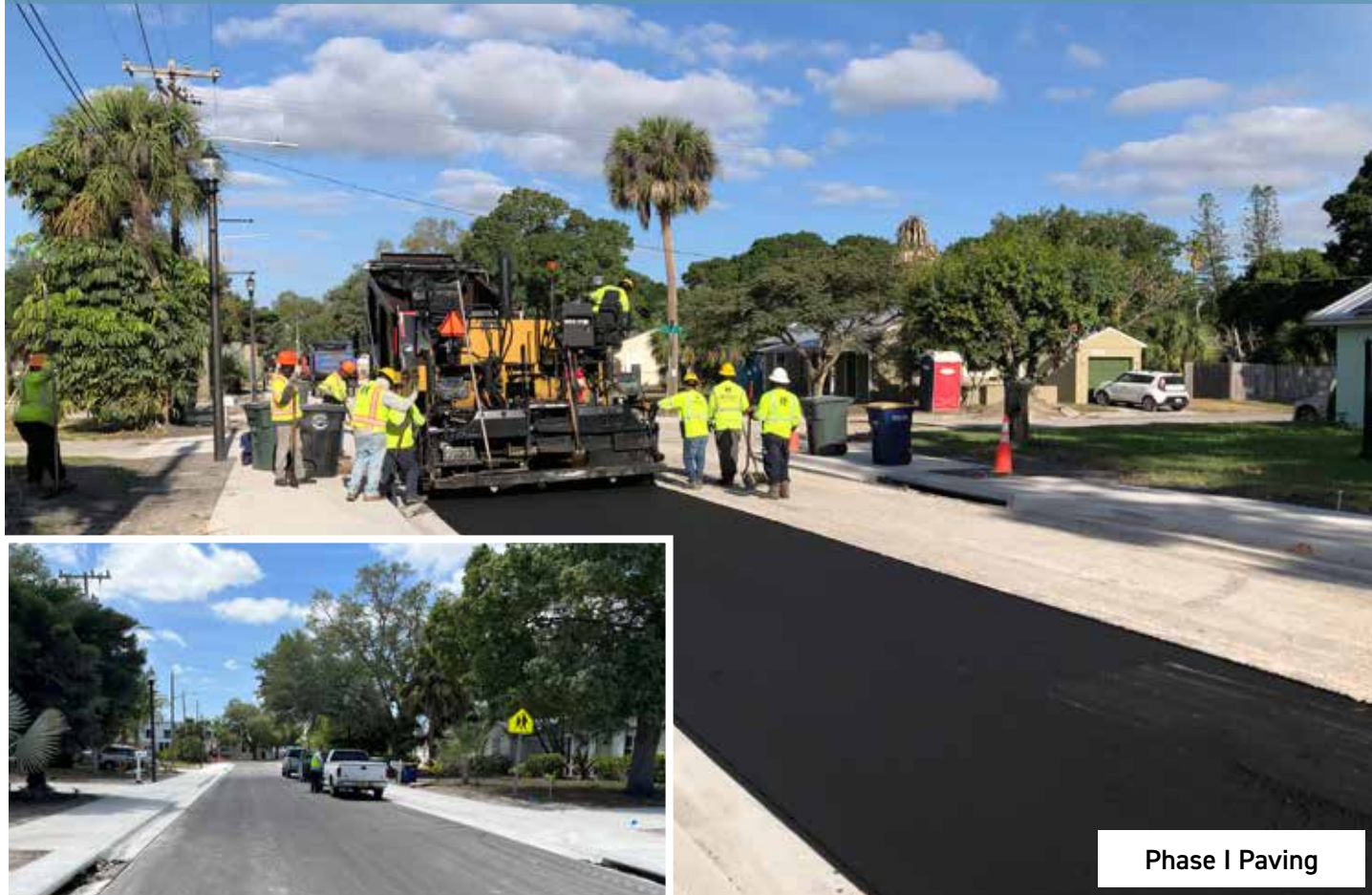
Phase I Lift of Asphalt
