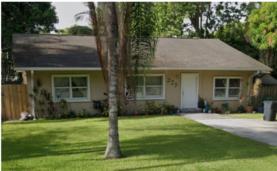
14. Re0120122sidence – Tumblin Kling Road – Facing South
