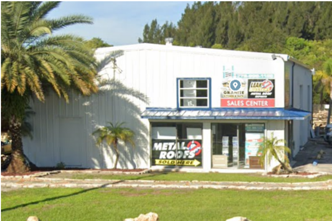
6. Leak Busters Roof Repair – Looking West – (ex. West side of US1, West of subject parcel)
