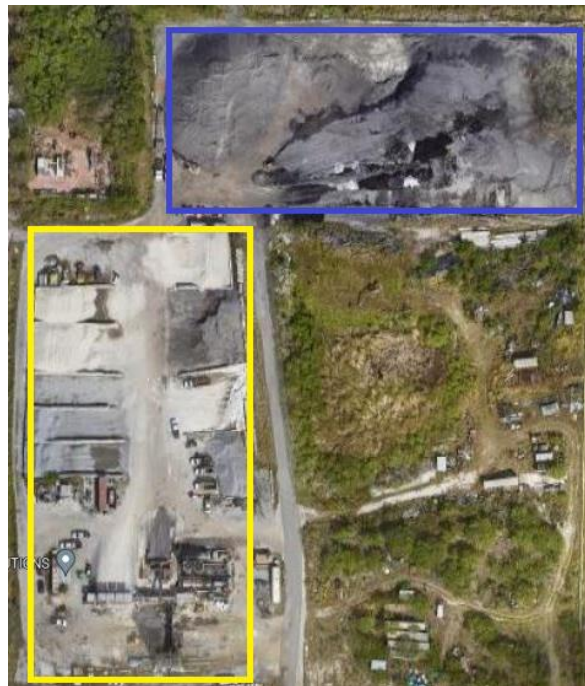
4060 Selvitz Road, Asphalt Plant
