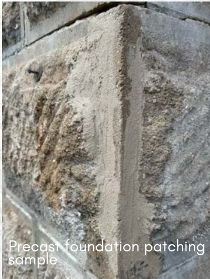
Precast patching sample
